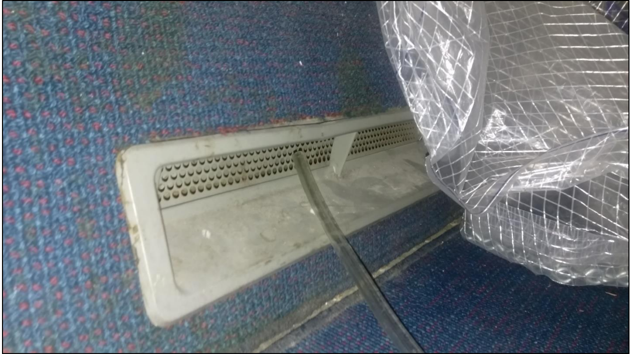
Figure 4.40 Vent Before ISOPASS, 737 Cabin
