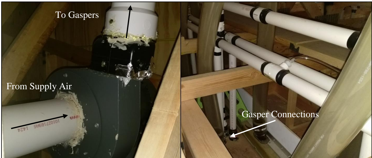
Figure 3.19 Boeing 767 Mock-up Supply Duct and Diffuser Connection (Patel, 2017)
