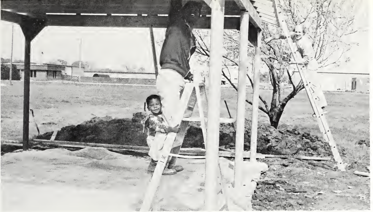
Andrew Galloway and daughter along with Pete Marchbanks work on the shelter house .
