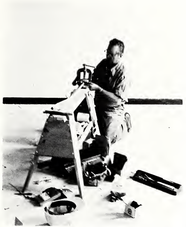
A physical plant employ preparing tubing for wire.
