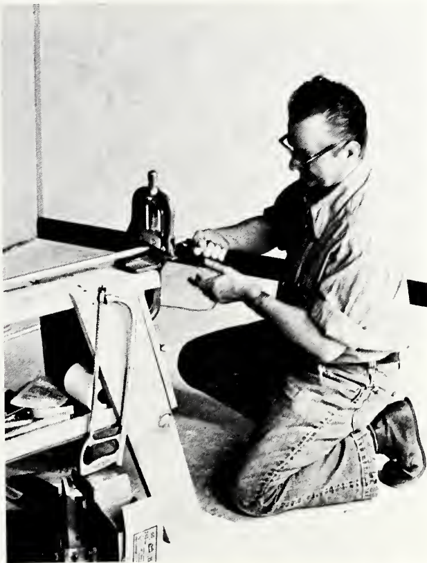
Henry Koskowski working on remodeling.
