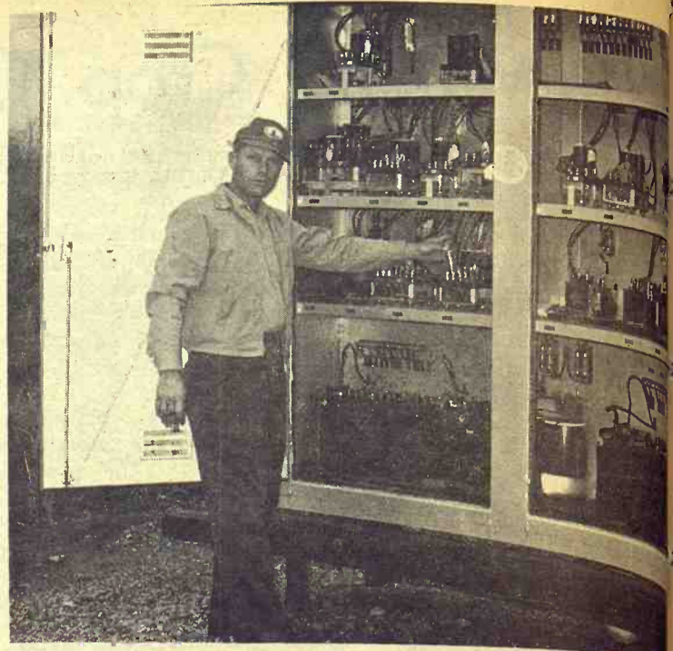
THE ARCOLA LINE MAN Ted Dinkel of Salina is a signal maintenance man for Union Pacific. He is shown here checking over automatic signalling equipment at Arcola, near Brookville. He maintains all signals and flasher crossings on UP mainline between Arcola and Solomon.
