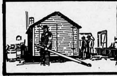
One Man Moves Buildings, Pulls Out Stalled Automobiles, Wagons, Tractors, etc.
