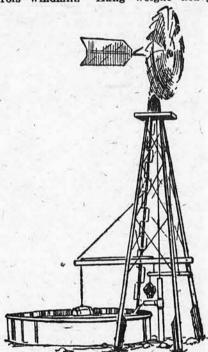
enough to pull mill out of gear when tank is full. Be sure to have float in tank several pounds heavier so when tank is low it will raise the weight on a level and release the windmill. F. S. Smith.
