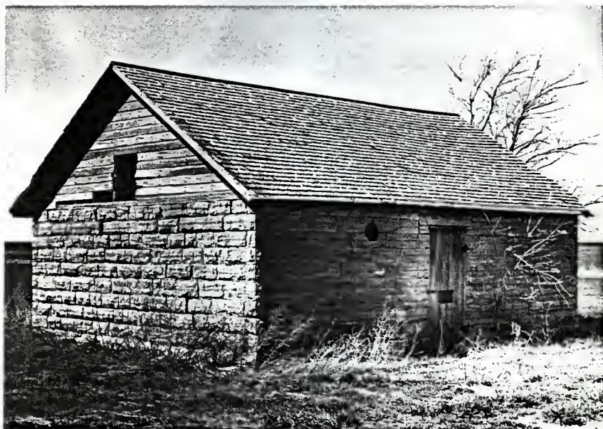
Fig. 5.42 Single-Crib Barn: Stone and Wood Construction
