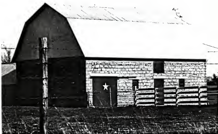
Fig. 5.52 Erie Shore Barn: Stone and Wood Construction and Gambrel Roof
