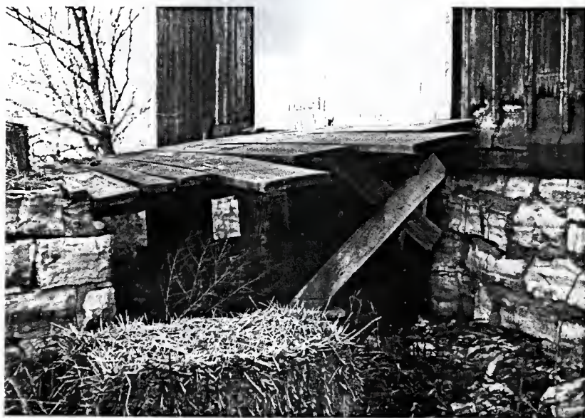
Fig. 5.24 Multi-level Barn: Wooden High Drive
