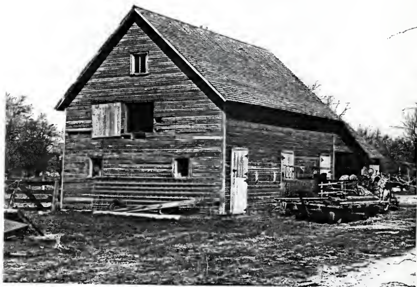
Fig. 5.8 Stable Barn: Gable Roof with End Addition
