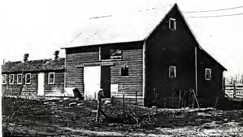
Fig. 5.35 English Barn: Wood Construction and Gable Roof
