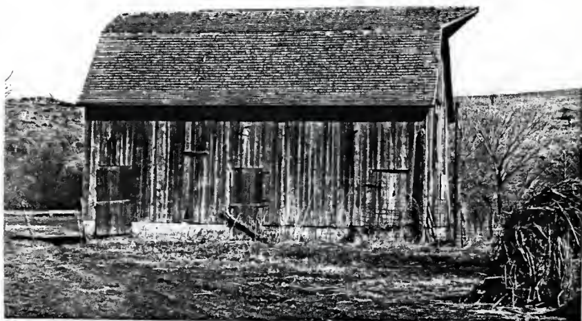
Fig. 5.10 Stable Barn: Gambrel Roof and Hay Hood
