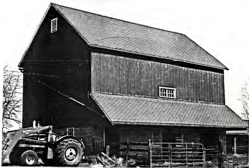
Fig. 5.31 Pennsylvania Dutch Barn: Pent Roof
