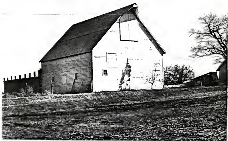
Fig. 5.4 Wisconsin Dairy Barn: Gable Roof
