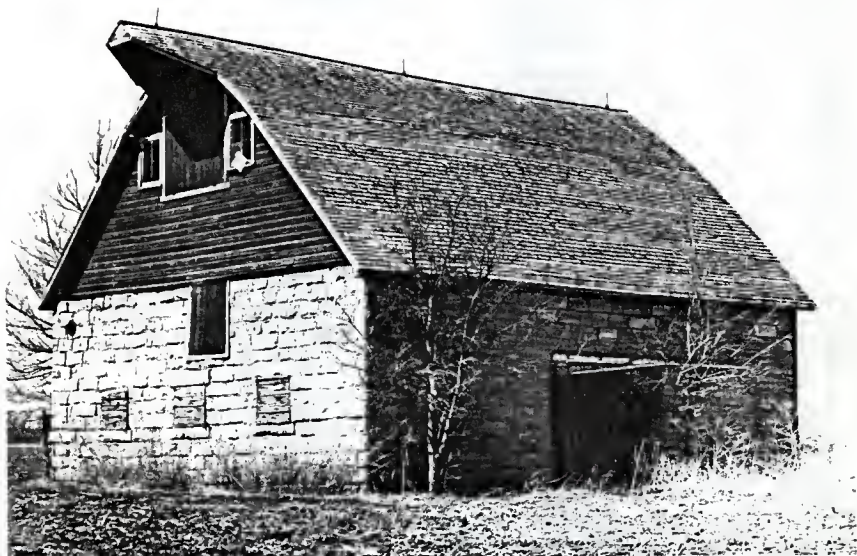
Fig. 5.37 English Barn: Stone and Wood Combination with a Gambrel Roof
