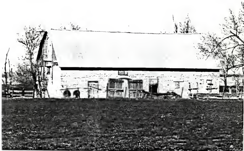
Fig. 5.53 Erie Shore Barn: End Extension Left of Drive-through
