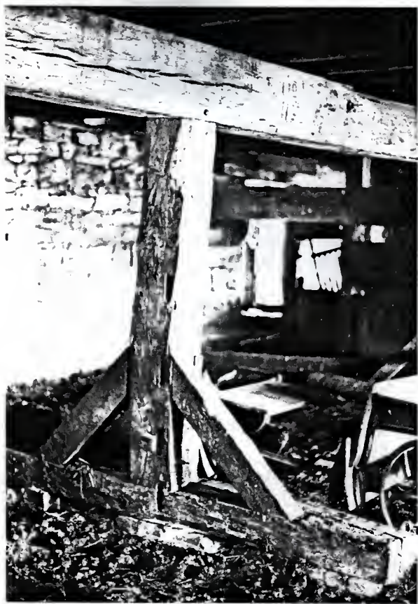
Fig. 5.30 Pennsylvania Dutch Barn: Newcomer Barn, Floor Sills
