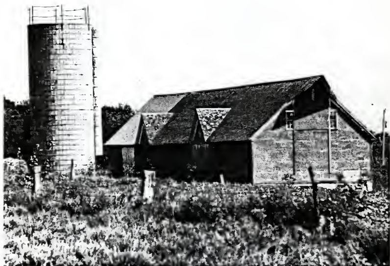
Fig. 5.22 Multi-level Barn: Upper Level Entrance
