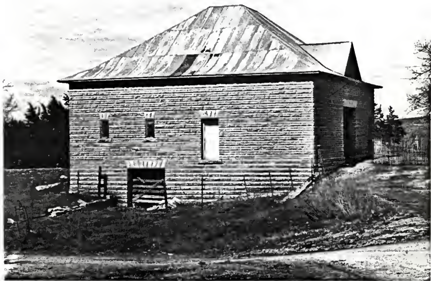
Fig. 5.67 Combination and Unclassified Barn: Stone Construction and Truncated Pyramid
