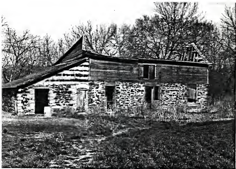
Fig. 5.9 Stable Barn: Stone and Wood Combination
