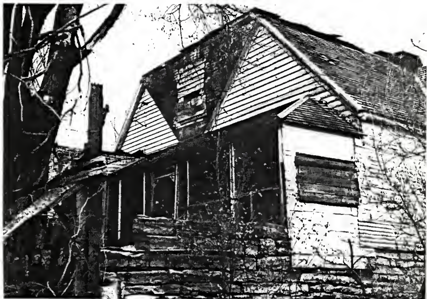
Fig. 5.58 Connected Barn: Shirley Barn, South Entrance to Residence
