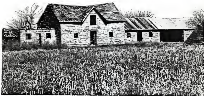
Fig. 5.61 Linear Barn: Stone Construction
