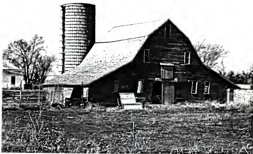
Fig. 5.16 Dutch Barn: Gambrel Roof with Side Additions
