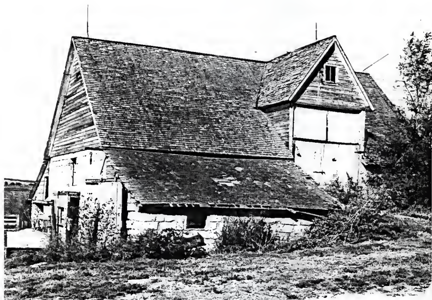
Fig. 5.66 Combination and Unclassified Barn: Stone and Wood Construction and Gable Roof
