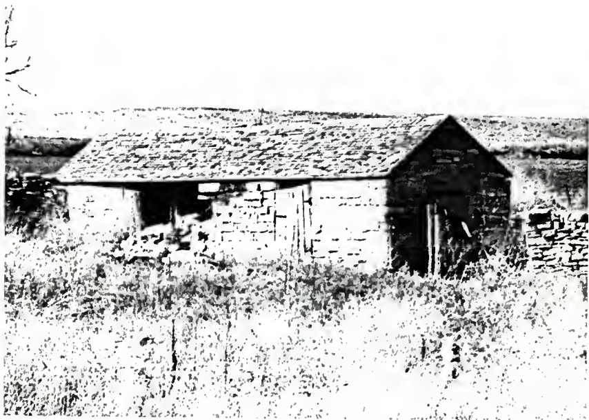
Fig. 5.41 Single-Crib Barn: Stone Construction
