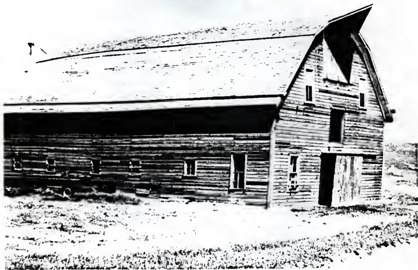
Fig. 5.15 Dutch Barn: Gambrel Roof
