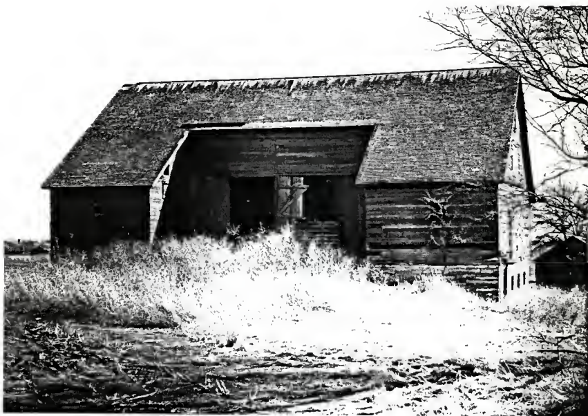
Fig. 5.29 Pennsylvania Dutch Barn: Newcomer Barn, North Elevation
