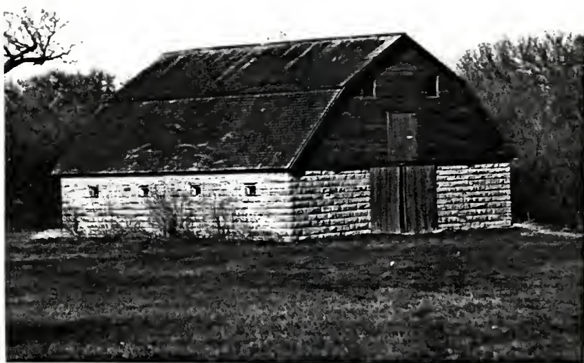
Fig. 5.18 Dutch Barn: Gambrel Roof with Stone and Wood Constuction
