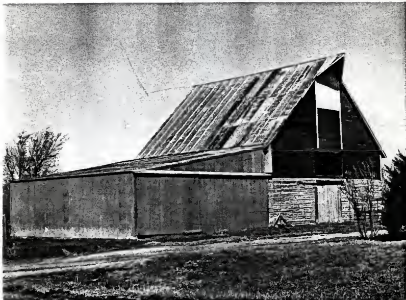
Fig. 5.17 Dutch Barn: Gable Roof with Stone and Wood Constuction
