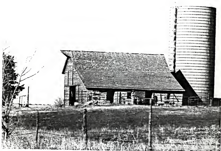
Fig. 5.48 Stable and Shed Barn: Hay Hood and Side Addition
