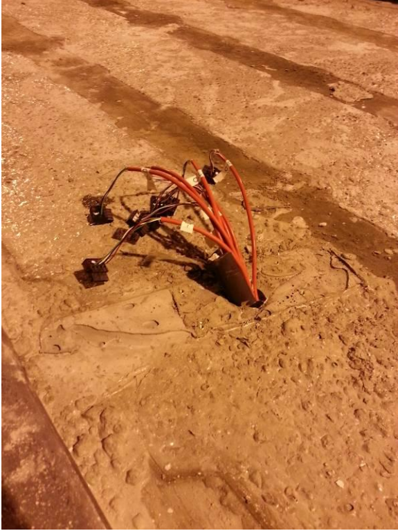
Figure 14.11 Wires exiting the crosstie after curing
