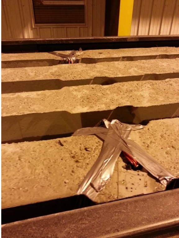
Figure 14.13 Wires taped before going through saw cutting process
