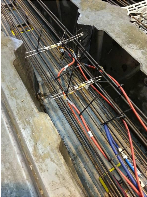
Figure 14.6 Gauges mounted at one end of a crosstie
