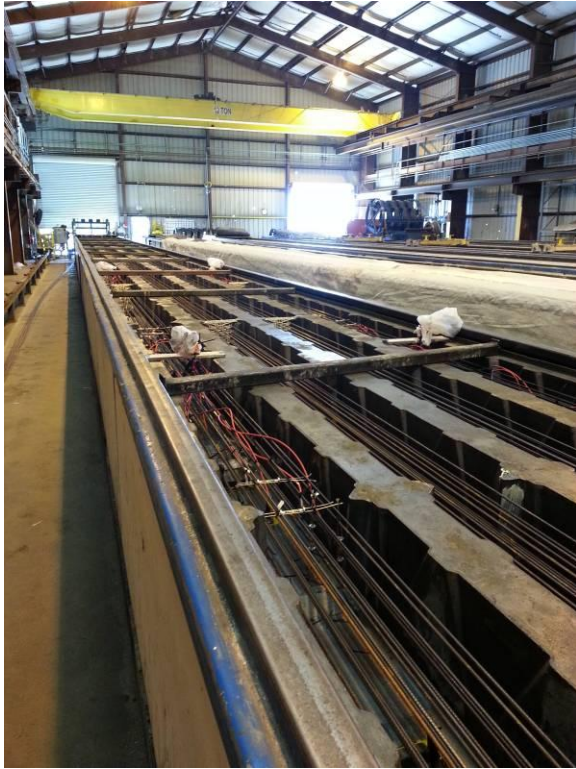
Figure 14.3 Crosstie forms with wire tensioned
