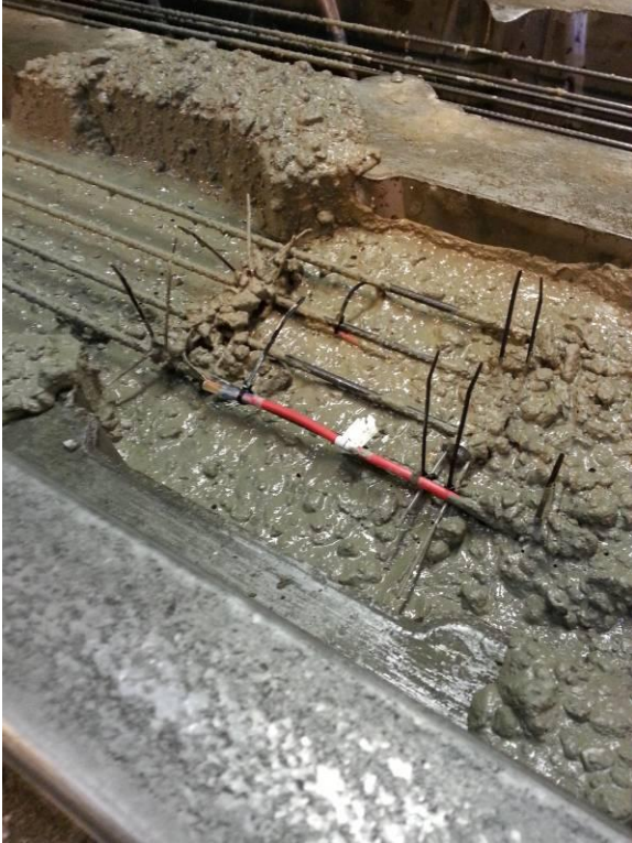
Figure 14.9 Crosstie being cast
