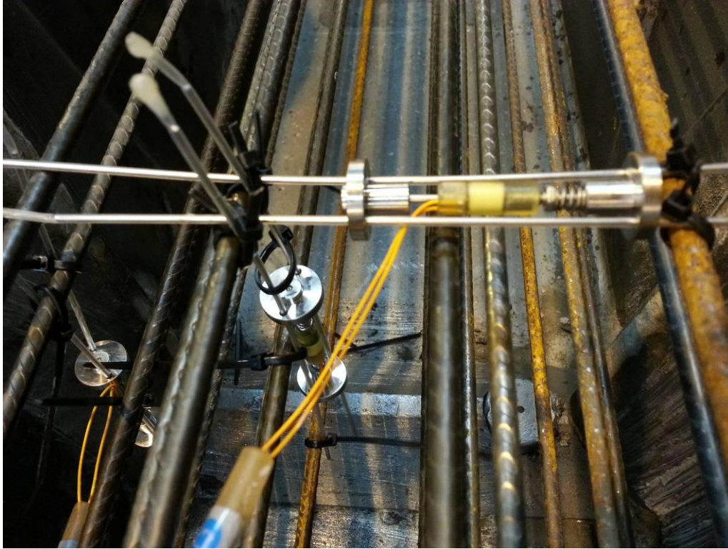
Figure 14.4 Close-up of gauges mounted to wires
