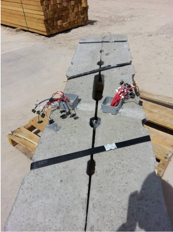
Figure 14.15 Crossties strapped to pallets and wire boxes installed
