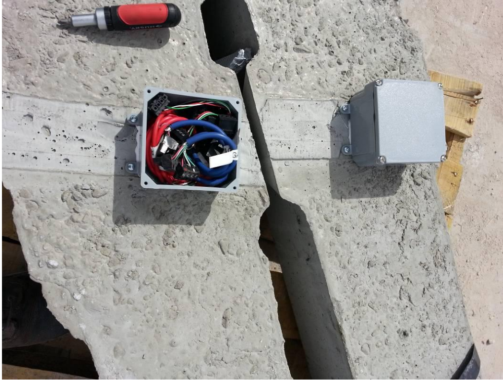
Figure 14.16 Wires placed into protective boxes
