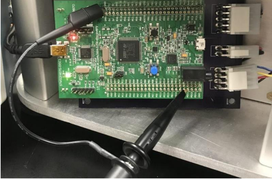
Figure 5.22 Control Loop Rate Verification using Oscilloscope
