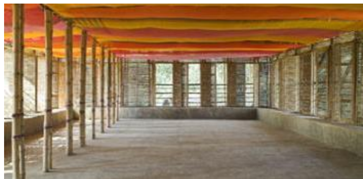
Figure 5-71 Upper floor of the school (Heringer, METI School, Bangladesh, n.d.)
