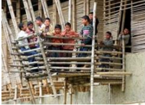
Figure 5-93 A small verandah on the upper floor (Lim, 2007)
