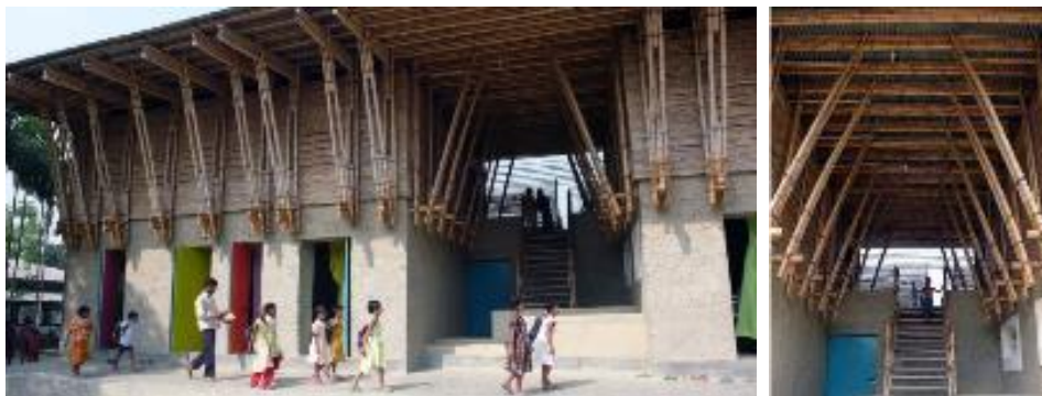
Figure 5-92 Bamboo stair of METI school links ground floor to upper floor (Lim, 2007)
