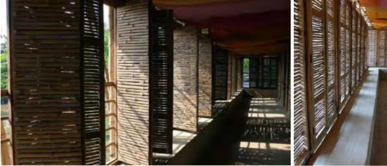
Figure 5-97 Upper Floor of the METI: Windows are made of bamboo (Lim, 2007).
