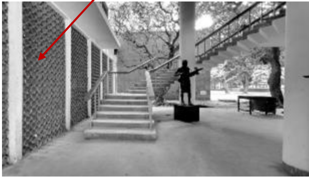
Figure 5-22 The terracotta screens made from traditional clay provide a degree of privacy (Earth, 2015)
