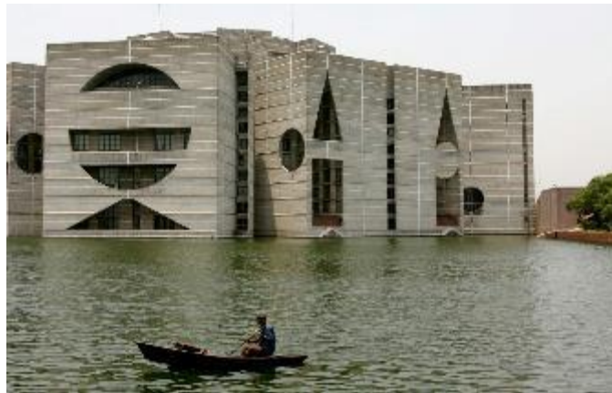
Figure 3-10 National Assembly Building, Dhaka: floating essence in the water (Islam, n.d.) One can realize that there are no real boundaries here between the Land and the River.
