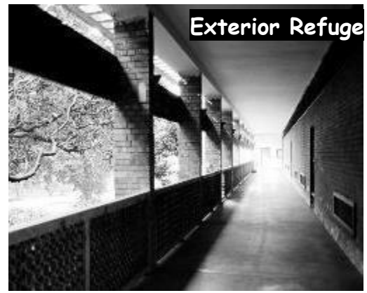
Figure 5-53 Upper floor corridor (Archive, n.d.)
