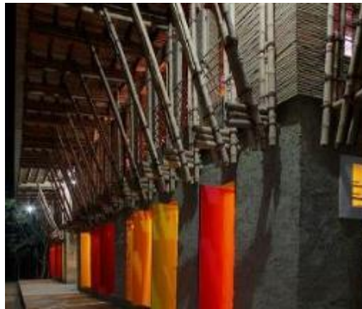
Figure 5-70 The exterior facade is punctuated with colorful doors and drapes (Hoerbst, n.d. )
