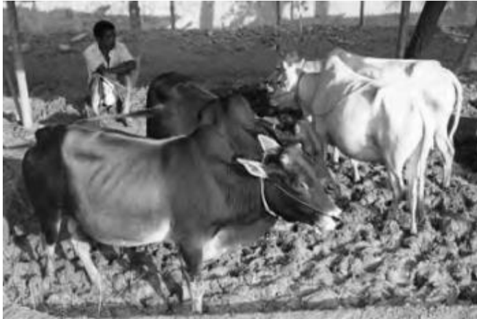
Figure 5-86 Use of Indigenous Methods: Cows are mixing loam, straw, and a little bit of water (Lim, 2007)
