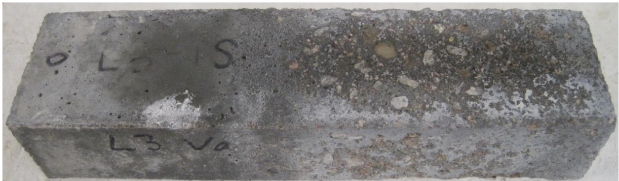
Figure 5.33: L3 Half-Immersed Concrete Prism
