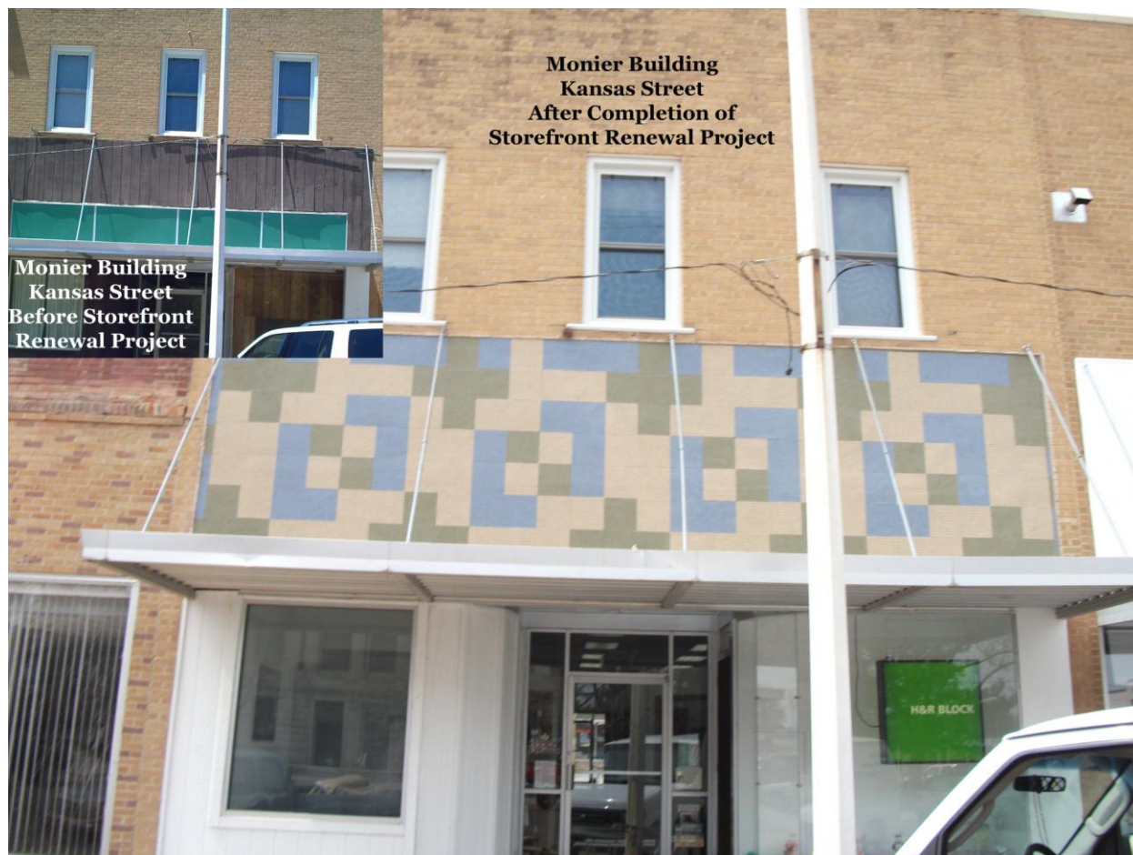
Figure 6.1 Storefront Renewal Project-2009: Monier Building-Kansas Street
