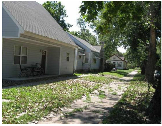
Looking towards south property
