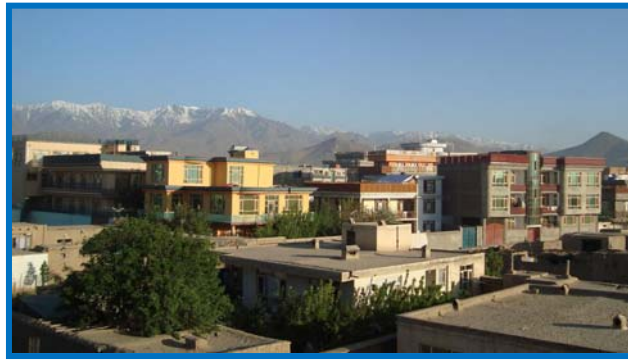
Figure3a. Houses in a neighborhood could be disturbed by an unethical architectural design. (Photo by the author)
