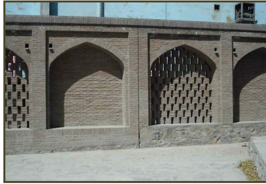
Figure 18a. A brick wall that shows variety of traditional patterns. (Photo by the author)
