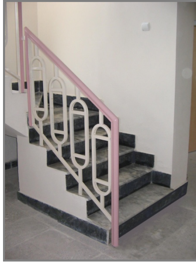
Figure12a. A staircase is an important connecting structural element of the house. (Photo by the author)
