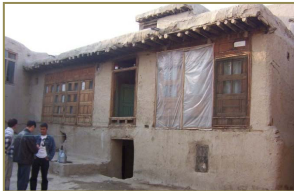
Figure 19j. Traditional overhang constructed to provide shade as well as to protect the house windows and outer mud walls from the rain. (Photo by the author)
