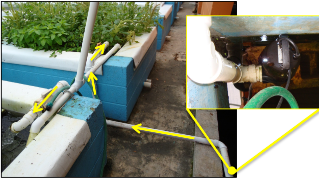
Fish tanks to plant tanks: water pump
