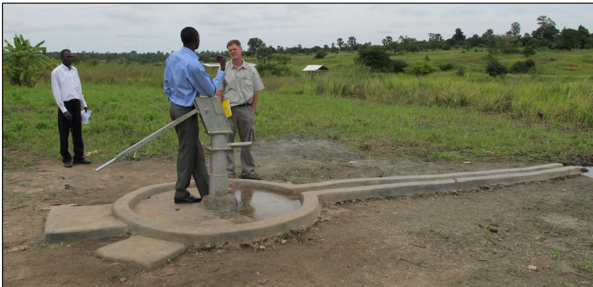
Figure 4.35 Typical Drilled Well in Gulu, Uganda
