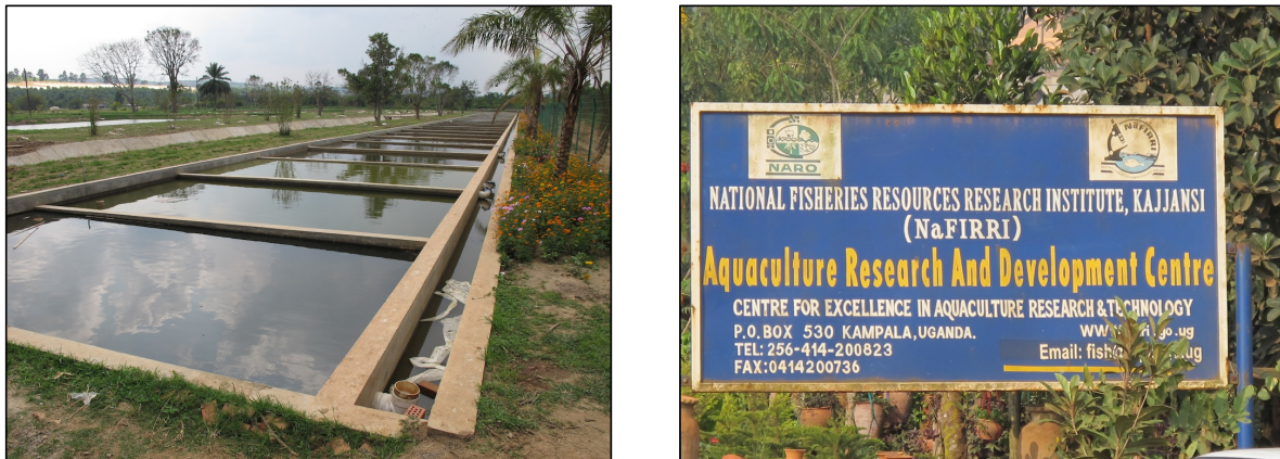
Figure 4.40 Kajjansi Aquaculture Facility Under Construction
