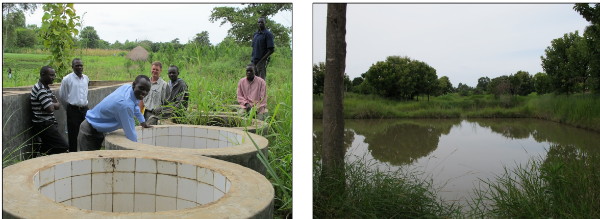
Figure 4.38 Failed Aquaculture Facility No. 2 in Gulu, Uganda
