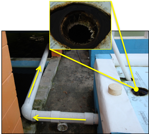
Plant tanks to fish tanks: gravity flow down standpipe
