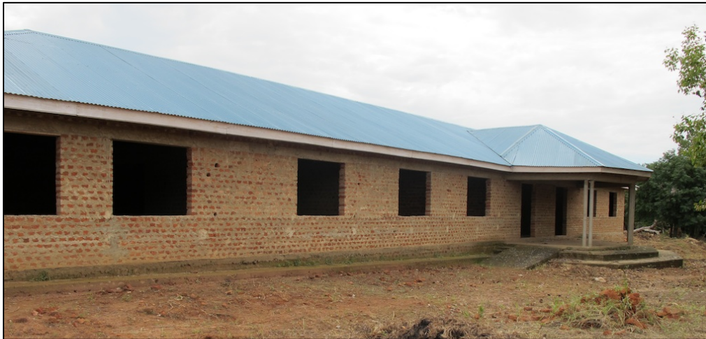
Figure 4.34 School Under Construction on Proposed Facility Site
