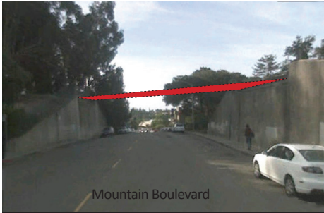
Figure 5.09 MontClair Rail Road Historic Overpass- Bridge Location Google Earth 2011
