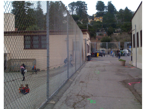
Figure 4.21 Fence Barrier on Terrace By Author 2011
