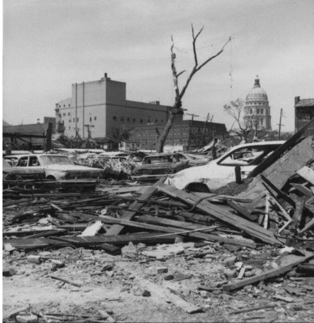
Figure 2-5 Destruction of 1966 Tornado
