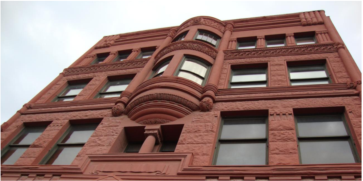
Figure 6-2, Columbian Building located on 6th street
