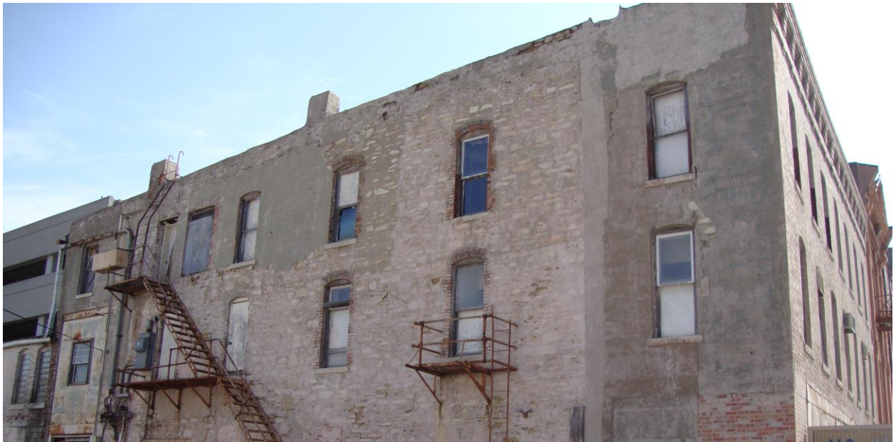
Figure 6-5 Building with only first floor usage
