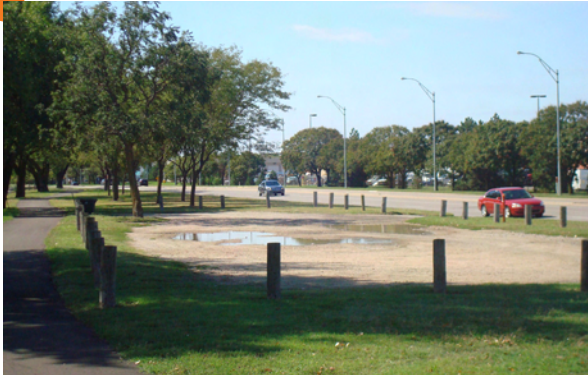
figure 3.18- gravel parking lot A gravel parking lot, in poor condition, is located along the riverfront across from City Maintenance facilities
