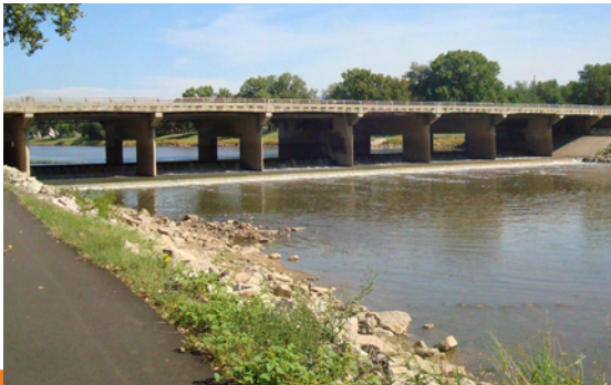
Figure 3.24- lincoln street bridge and dam
