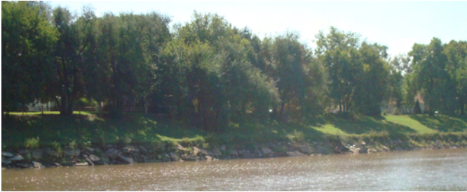
figure 9.11- rip-rap along river's edge
