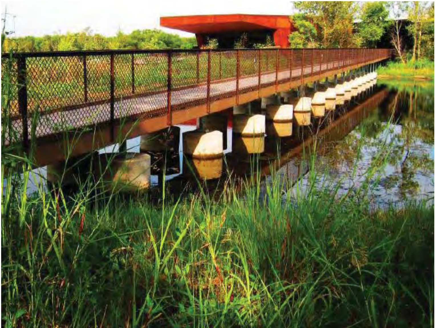
Figure 5.45- bridge over wetlands to audubon center
