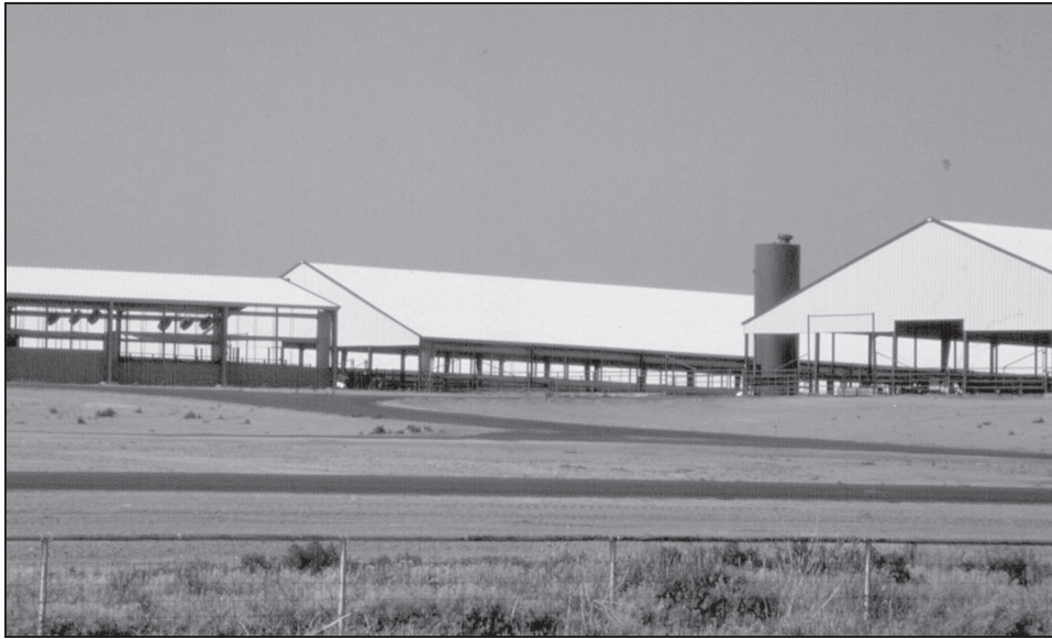
FIG. 8—The open sides that characterize most freestall barns, including these at the Santa Fe Dairy in Grant County, Kansas, provide ventilation. (Photograph by David Kromm, June 2004)
