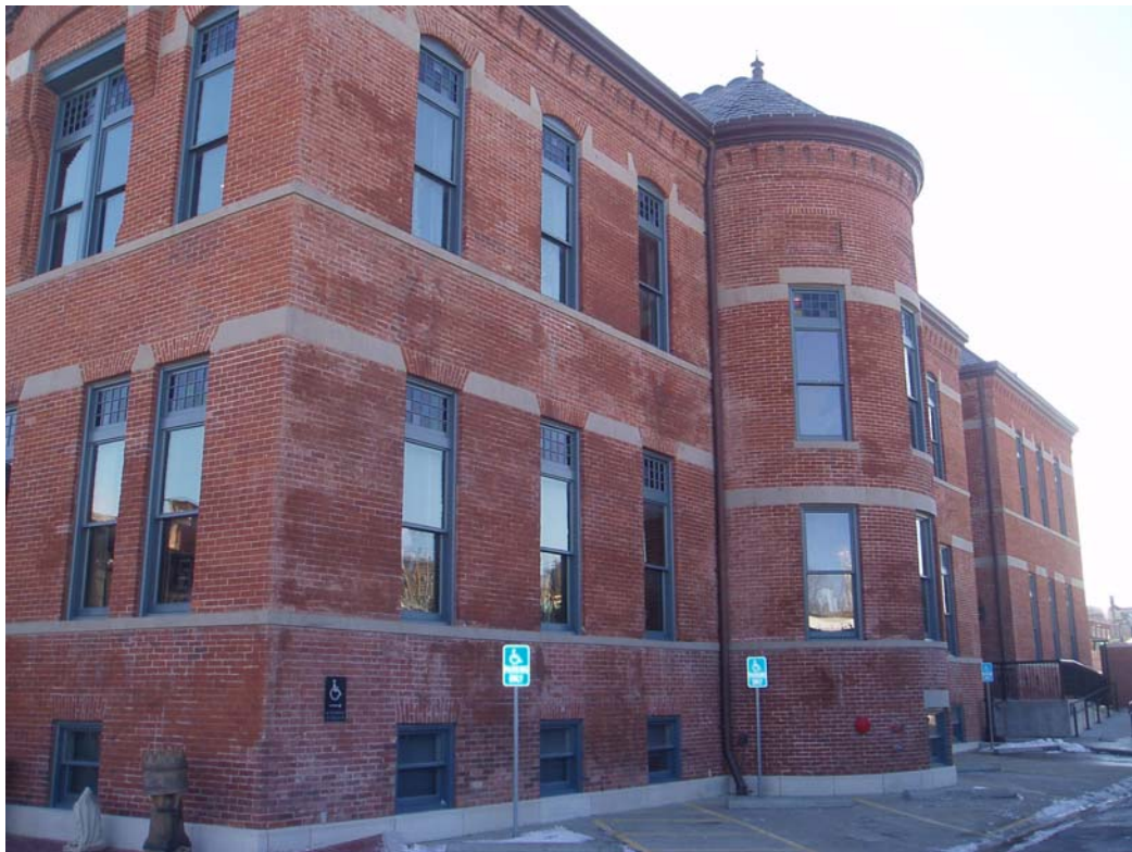
Figure 53. Side view of the Webster House exterior
