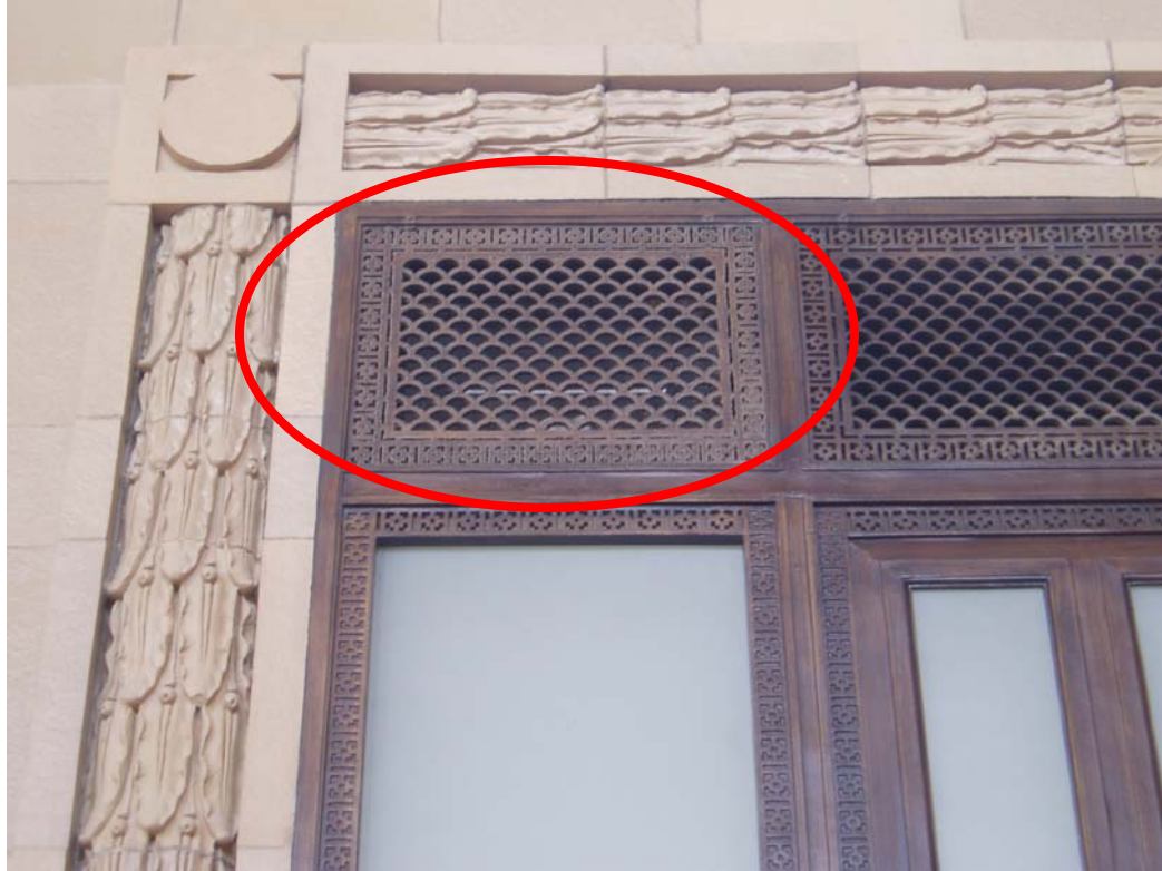
Figure 30. Location of speakers for the fire and evacuation annunciation system
