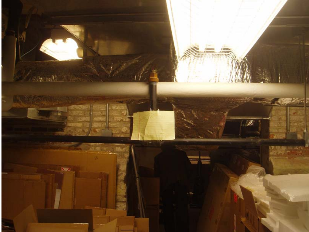
Figure 61. Basement mechanical room
