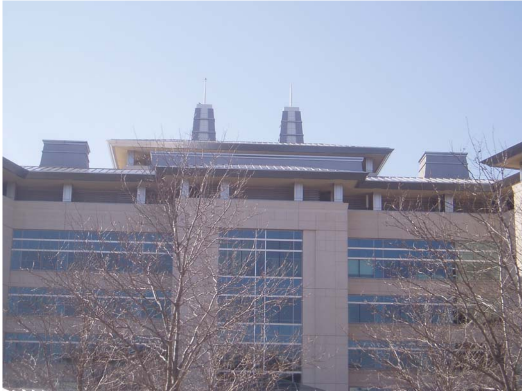
Figure 8. Penthouse roof level
