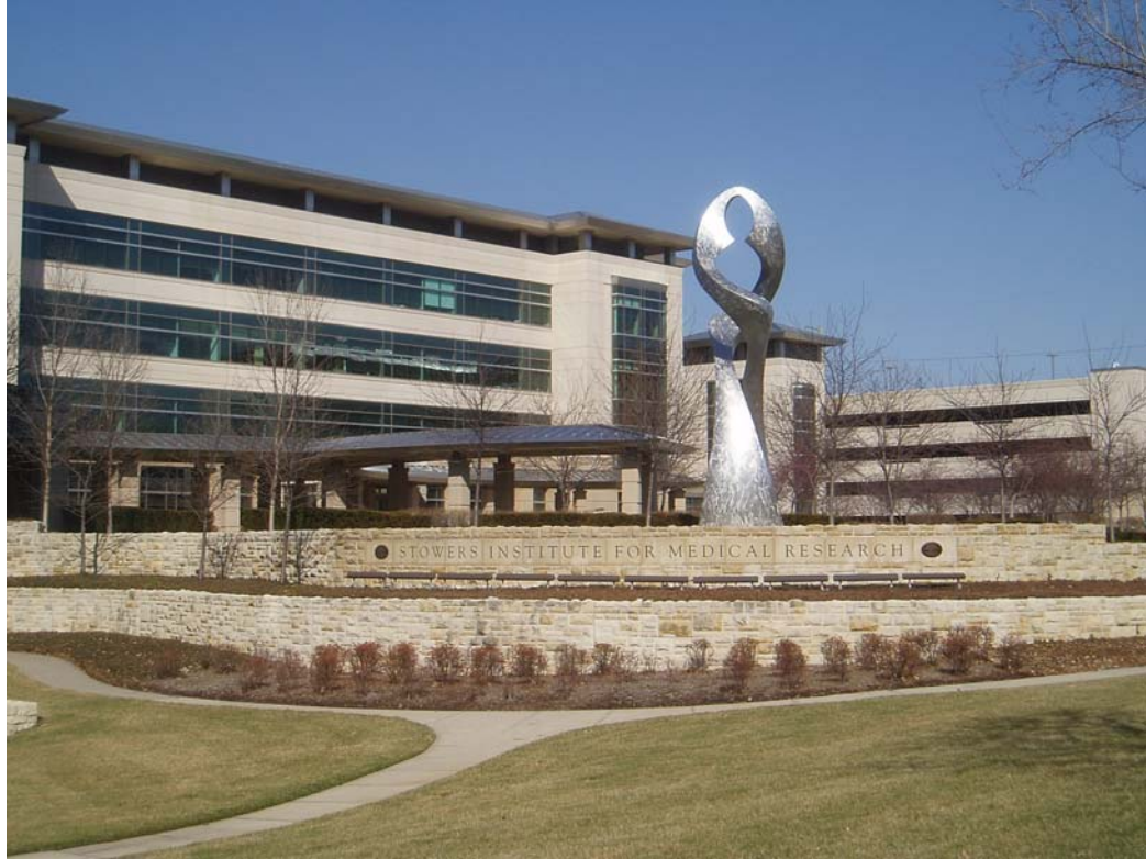
Figure 6. Stowers Institute campus buildings
