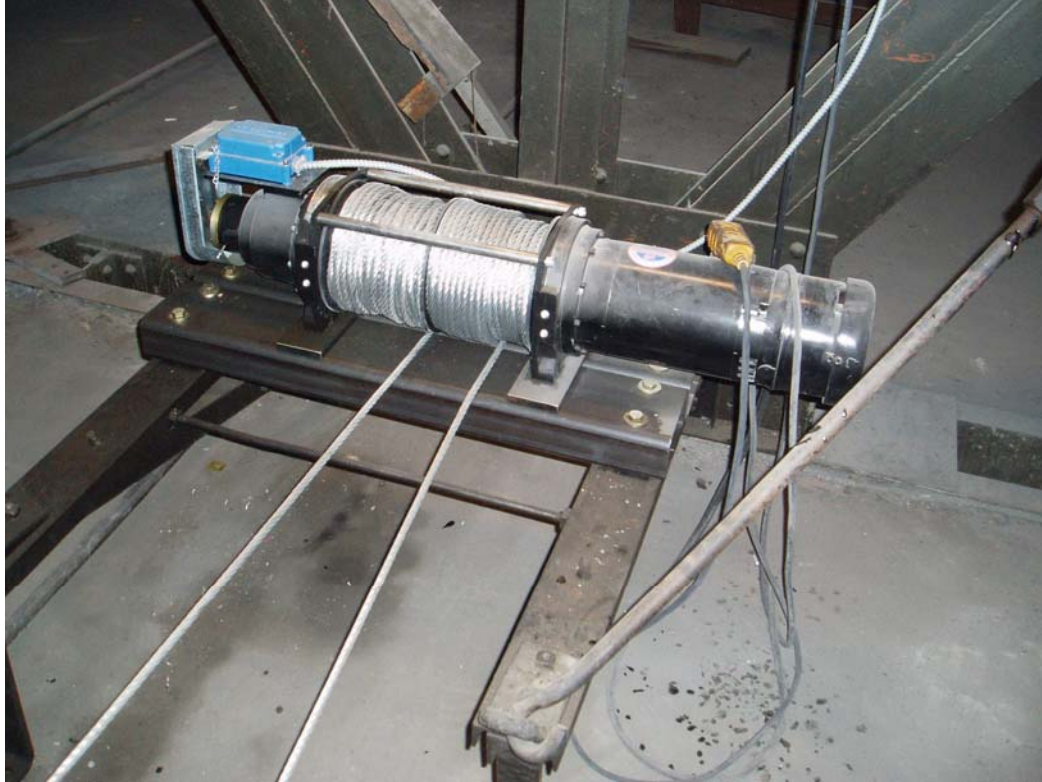
Figure 38. The chandeliers' new pulley system
