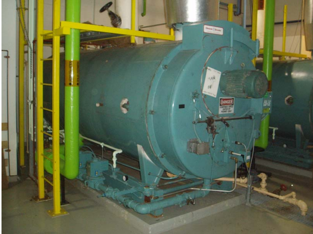
Figure 12. Steam boiler
