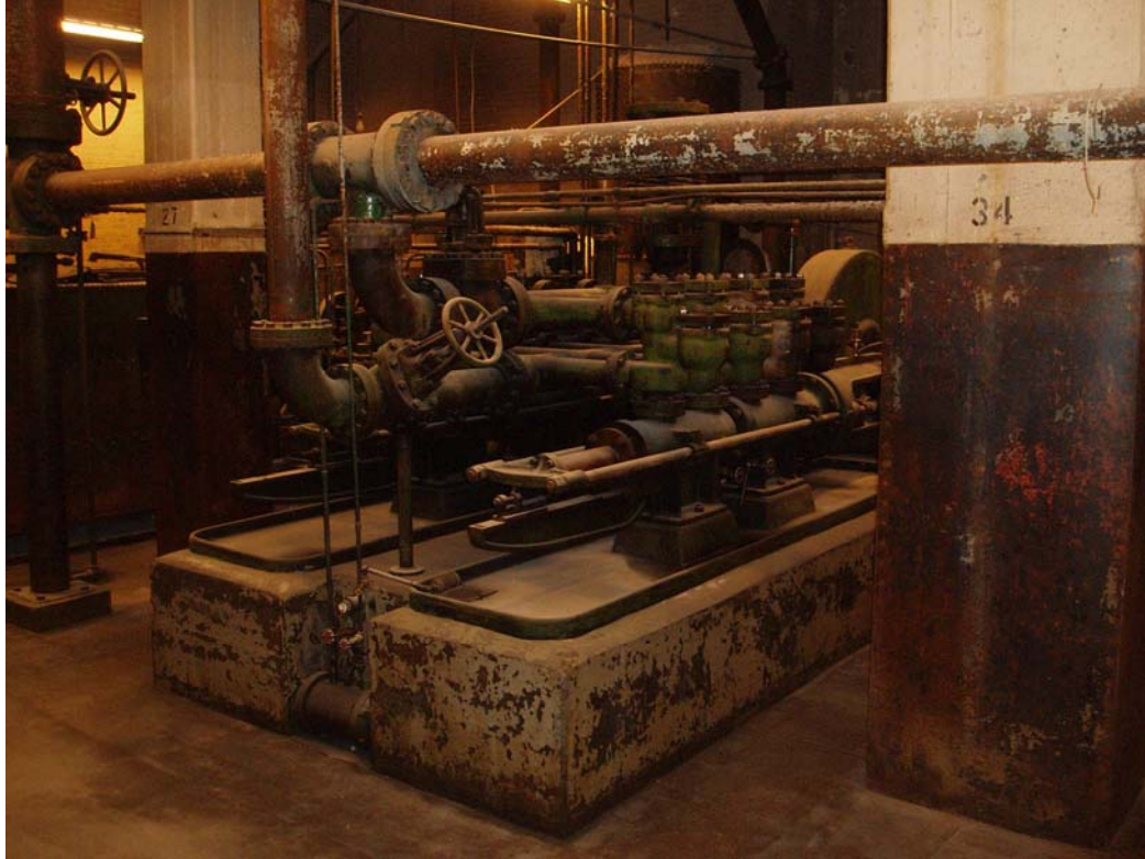
Figure 25. Historic Union Station chiller and valves
