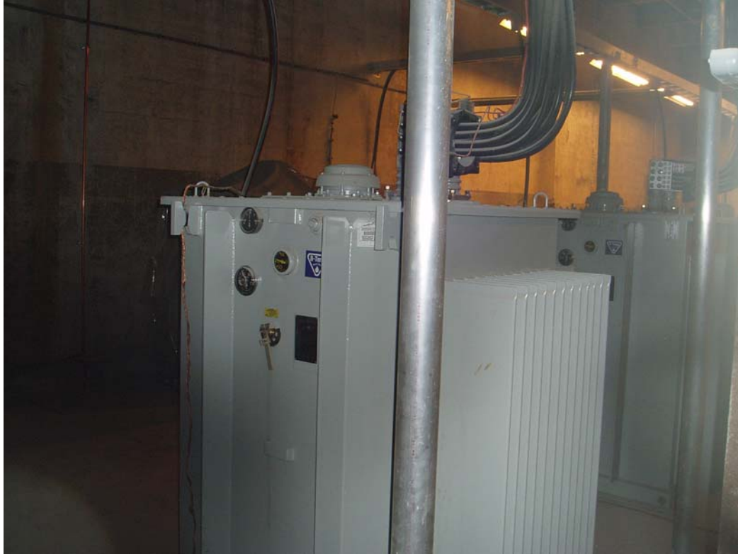
Figure 44. A typical transformer
