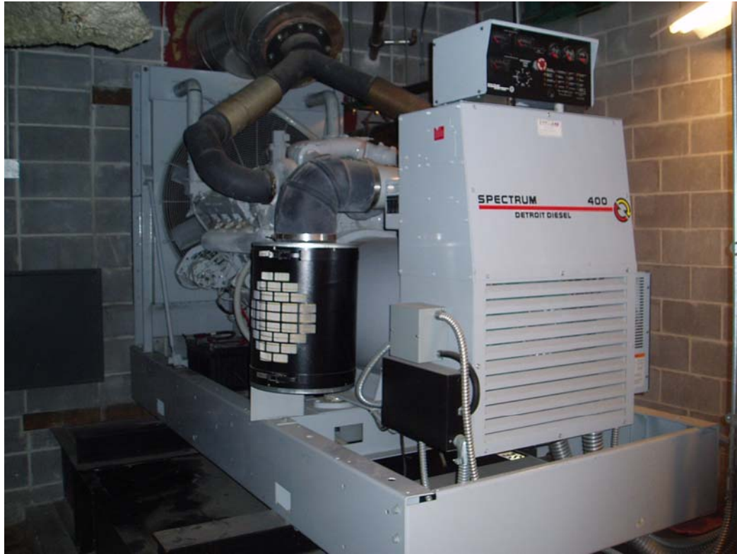
Figure 46. Emergency power back-up generator
