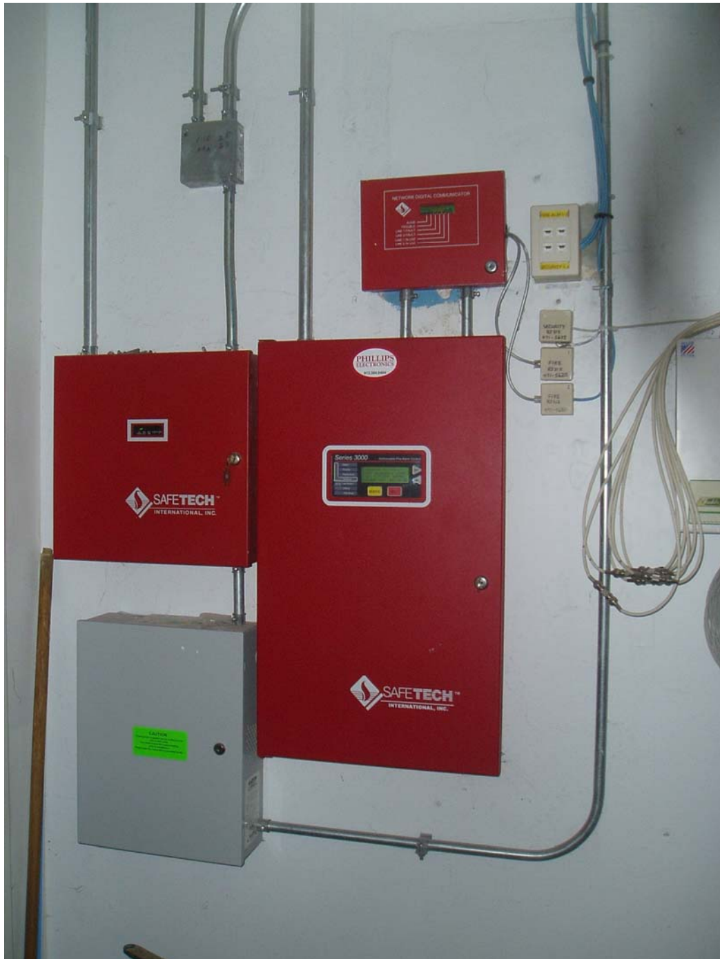
Figure 64. Main fire panels
