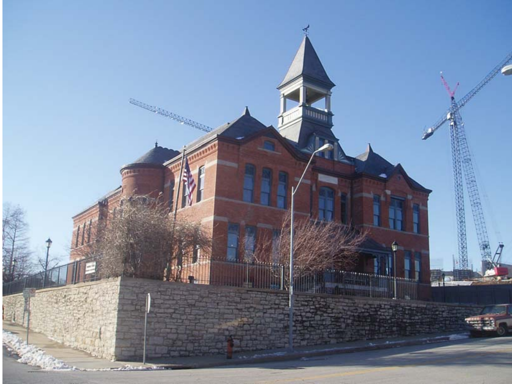
Figure 49. Exterior of the Webster House
