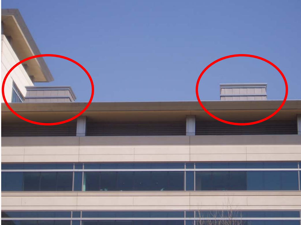
Figure 9. Exhaust penetrations through the roof
