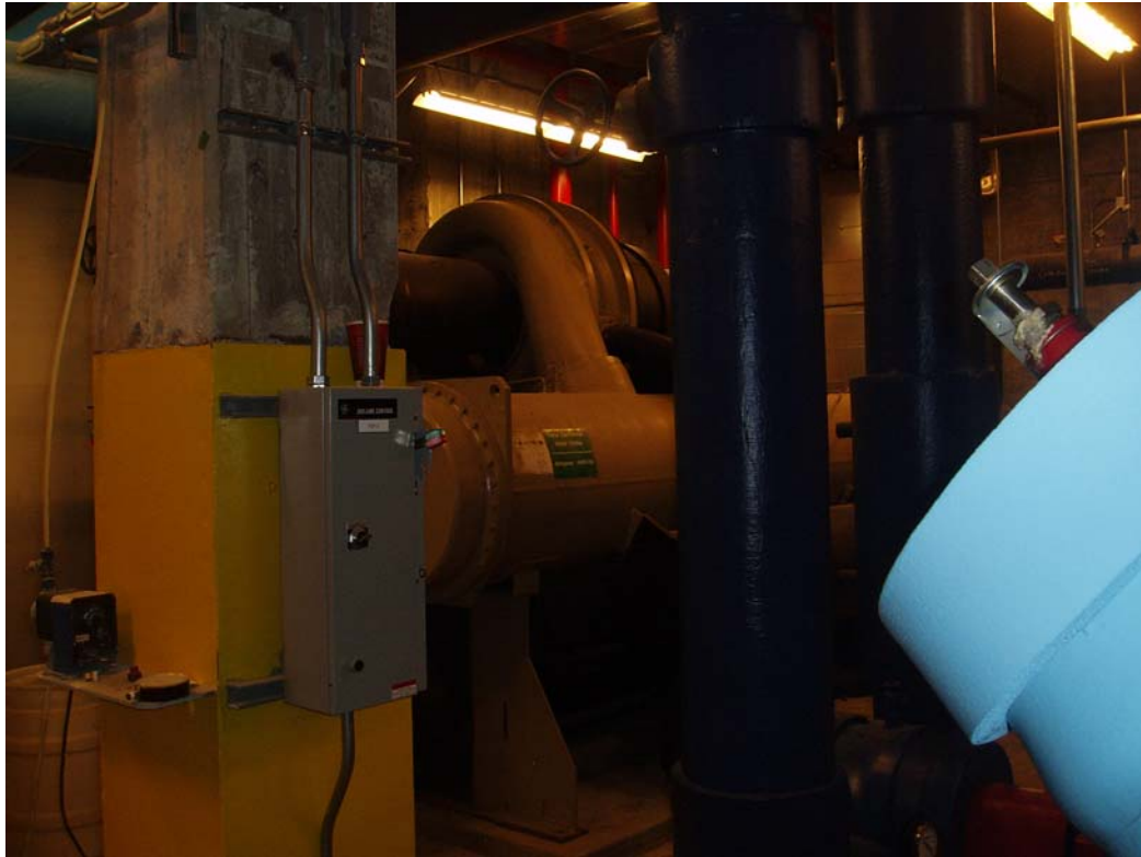
Figure 27. Union Station chiller
