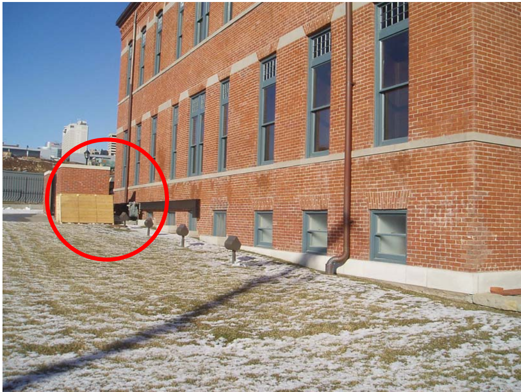
Figure 59. The grease interceptor is located outside of the building and behind brick walls
