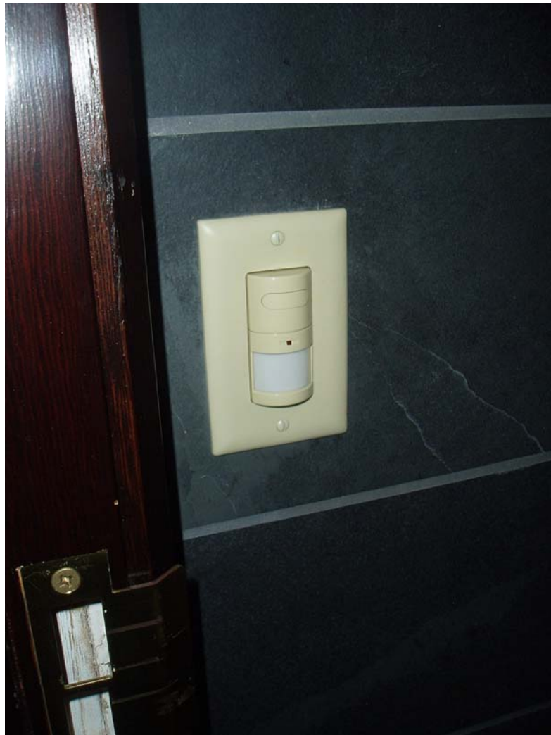
Figure 63. A motion sensor
