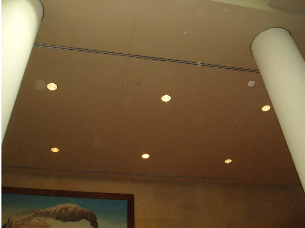
Figure 47. Track lighting above the stairs
