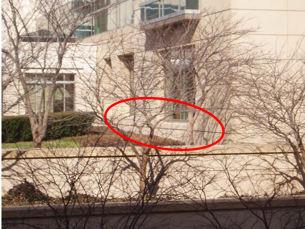
Figure 10. Outside air intakes along the building perimeter.
