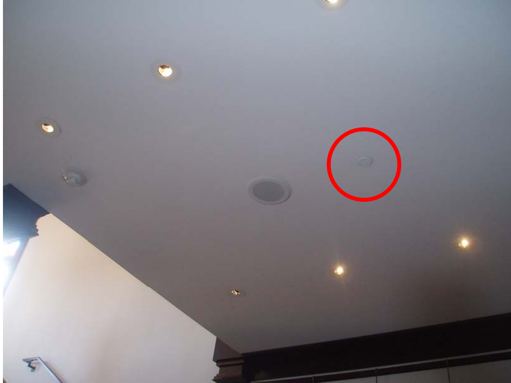
Figure 65. Interior room ceiling and recessed sprinkler heads
