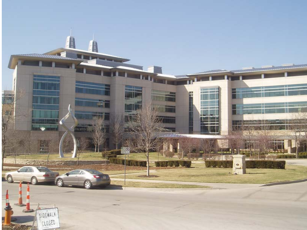
Figure 7. Exterior band of windows
