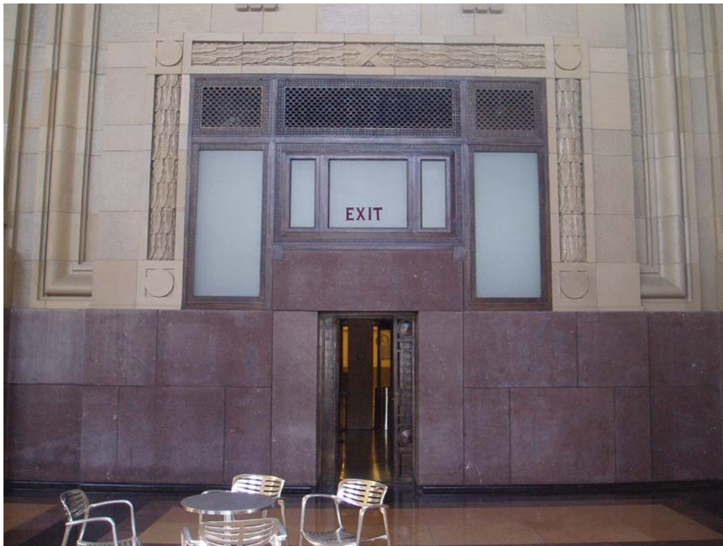
Figure 41. North waiting room exit signs
