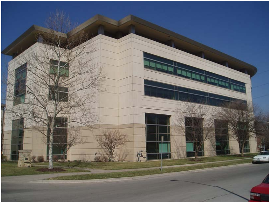
Figure 4. Four-story administrative building
