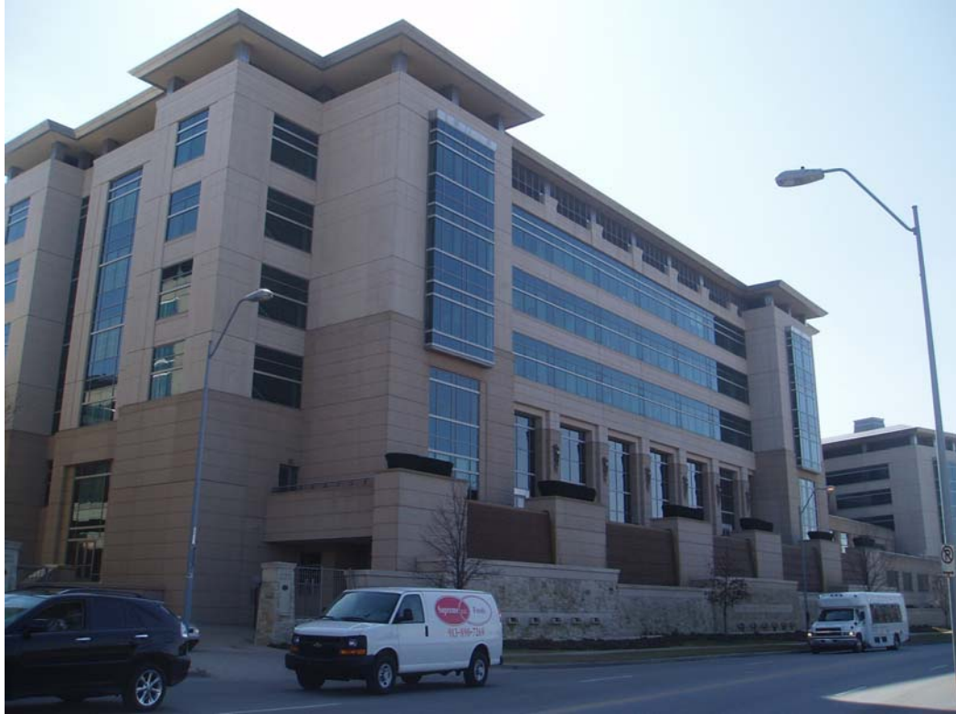
Figure 3. Six-story research building complex
