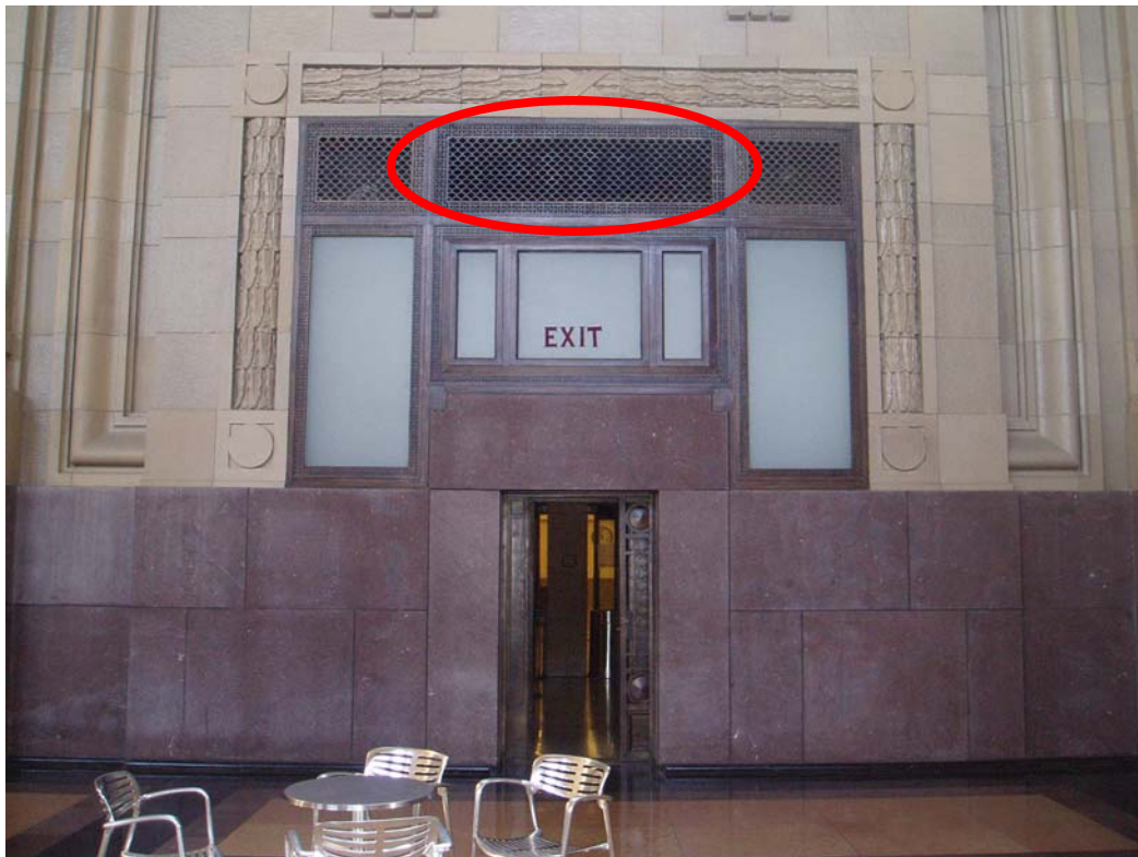
Figure 29. Supply air grills
