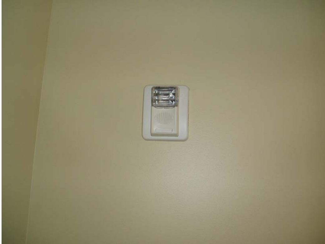
Figure 66. Fire notification device
