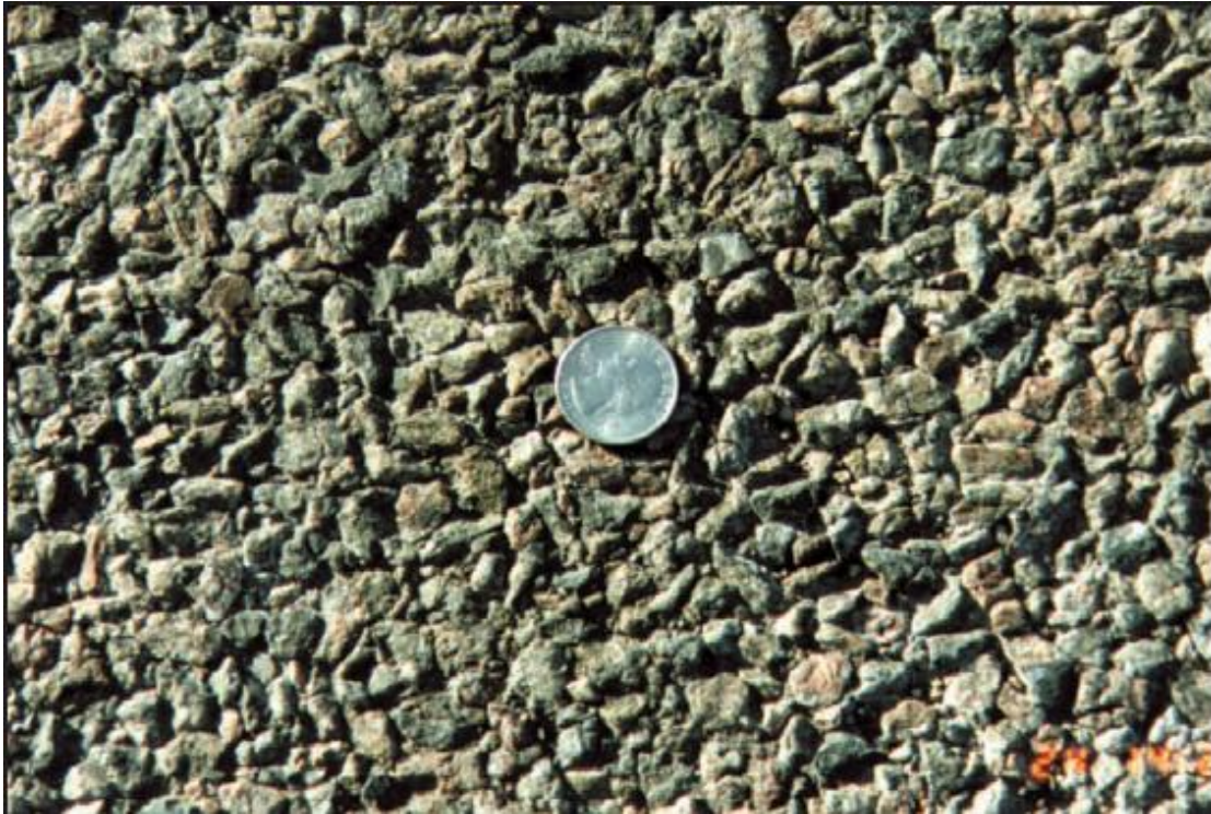
Figure 2.8 Chip Seal Constructed with Single-Size Aggregates (Wood et al. 2006)
