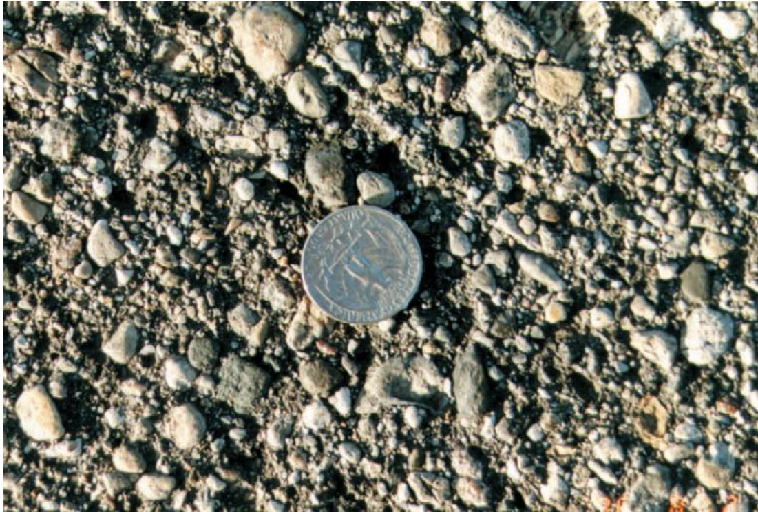
Figure 2.9 Chip Seal Constructed with Graded Aggregate (Wood et al. 2006)
