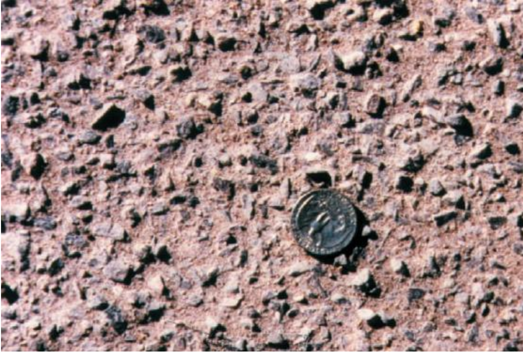
Figure 2.13 Chip Seal Constructed with High-Dust-Content Aggregates after Sweeping (Wood et al. 2006)
