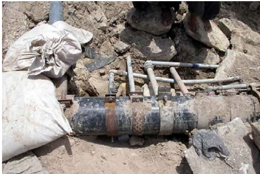
Water/wastewater infrastructure are often illegally tapped, exposed, or have leaks which introduce disease into the community. Source: Bechtel Corporation, 2003.
