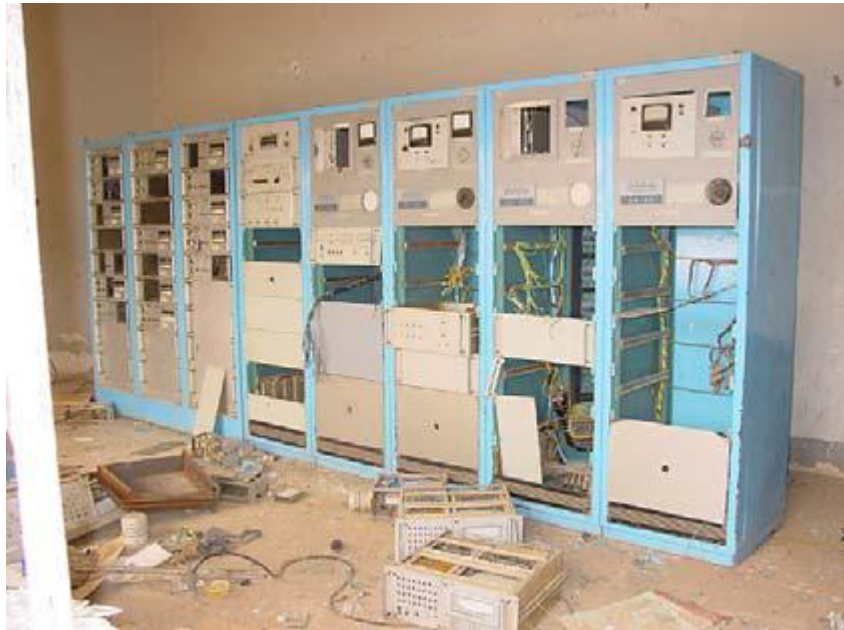
Iraq power infrastructure has been the target of destruction and looting, such as this Substation Control System. Source: Bechtel Corporation, 2003.
