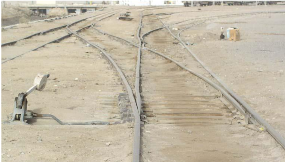
Kinks in the railroad system network are common. Iraq struggles to keep railroad materials from being looted and the network itself maintained. Source: Bechtel Corporation, 2003.
