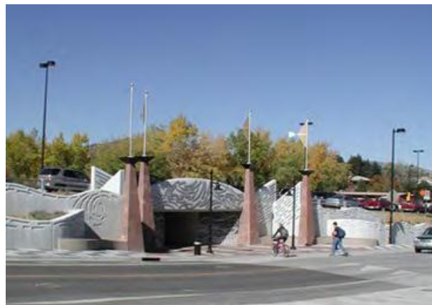
Figure 5.1. Bicycle and pedestrian underpass in Boulder, Colorado (LSA Associates Inc., 2008).
