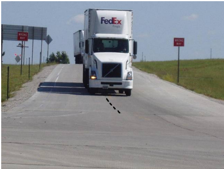
Figure 3-11 Ramp Before Final Striping at I-35/US-75 Interchange
