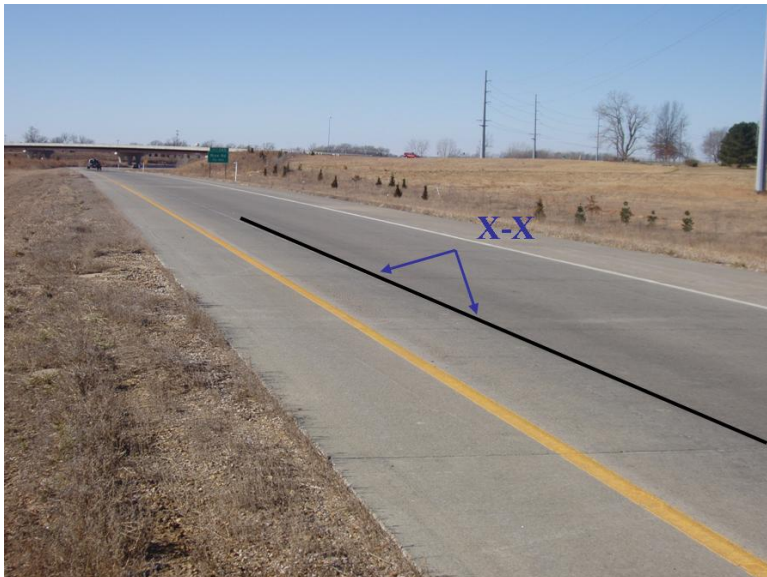
Figure 3-10 Configuration of the Joints and Pavement Markings at the K-4/KTA Interchange
