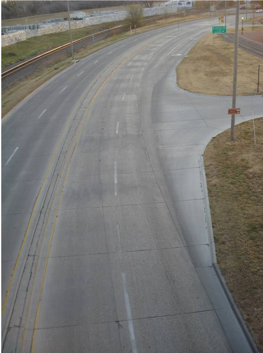
Figure 3-8 Condition of Newly Applied Pavement Markings at Ft. Riley Blvd.
