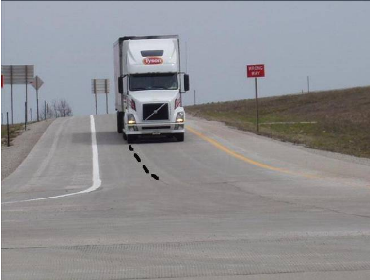
Figure 3-12 Ramp After Final Striping at I-35/US-75 Interchange
