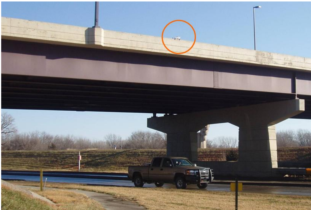
Figure 3-7 Security Camera on Kansas River Bridge at the Test Site (Second Stage)
