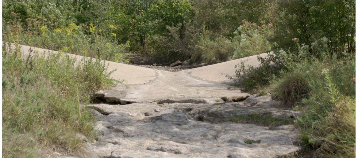
Figure 2.10. Steams flow measurement station using a v-notch weir at Kings Creek
