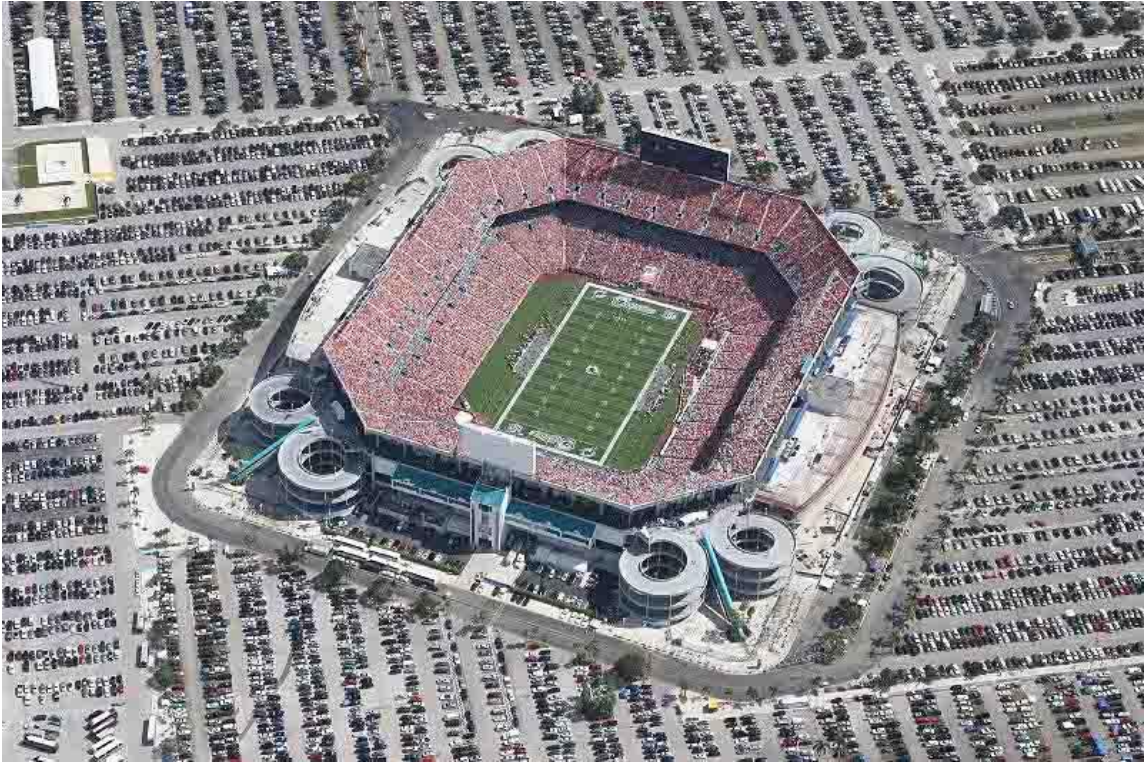
Figure 5-2, Dolphin Stadium - Miami Florida.
