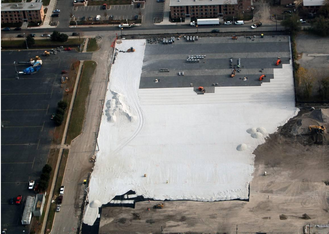
Figure 3-29, Construction Photograph – Lot ‘L’ US Cellular Field, (Site Design Group, Ltd., 2009).
