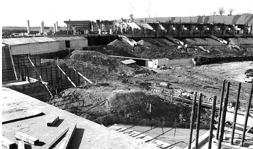
Figure 4-1, Construction Photograph, Truman Sports Complex (Lewis, 1977, p. 81)
