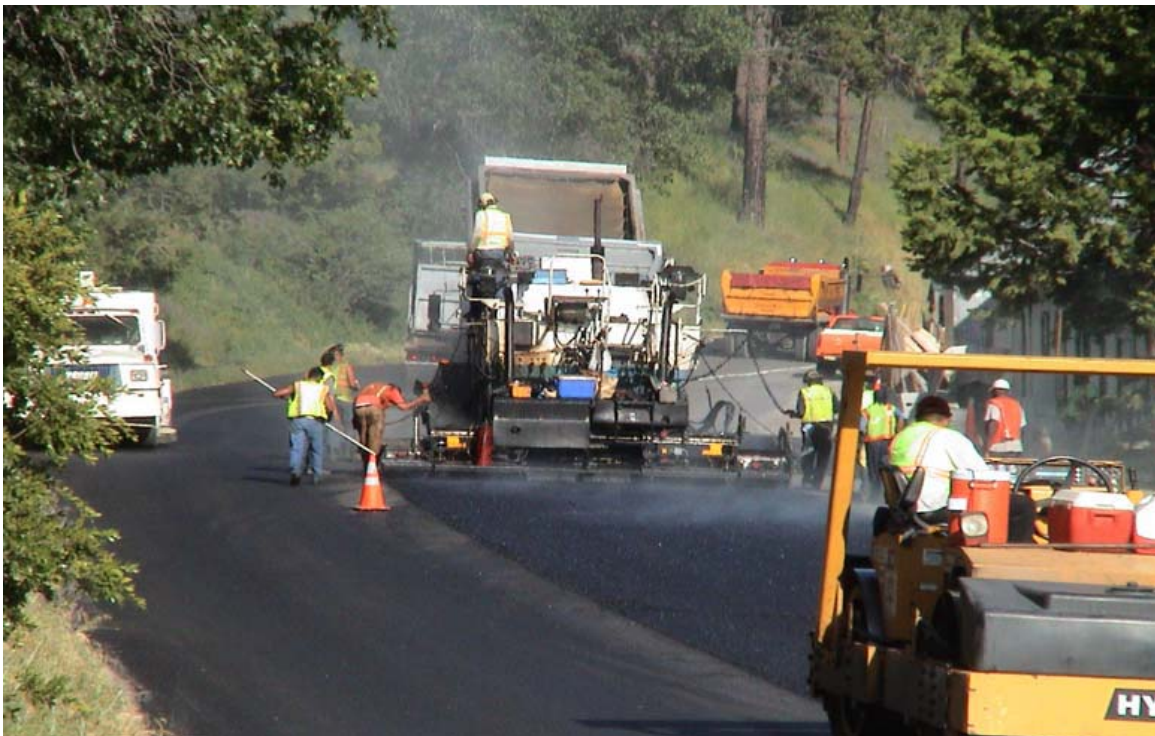
Figure 2-8 Roller Position during Nova Chip Application (Caltrans, 2003)
