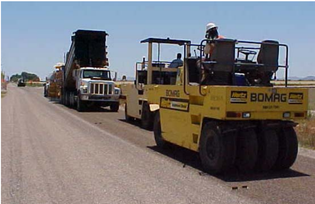
Figure 2-14 Pneumatic (Rubber-Tired) Roller (Caltrans Division of Maintenance, 2003)
