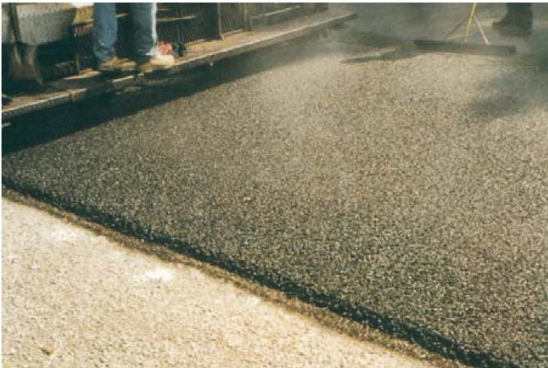
Figure 2-7 Freshly Laid Nova Chip (Caltrans, 2003)
