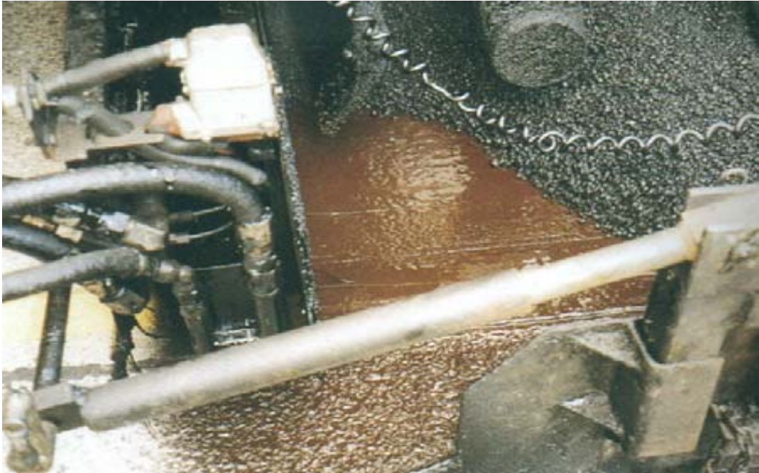
Figure 2-6 Emulsion Membrane and HMA Mix Spreading (Caltrans, 2003)
