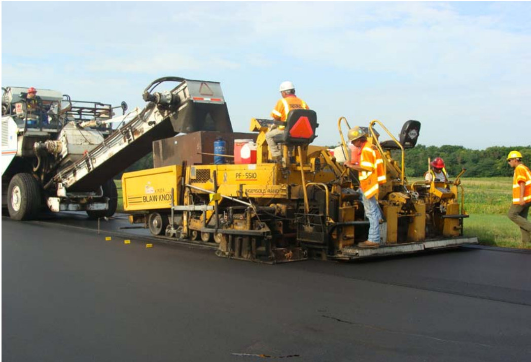
Figure 2-3 Application of thin HMA by Asphalt Paver
