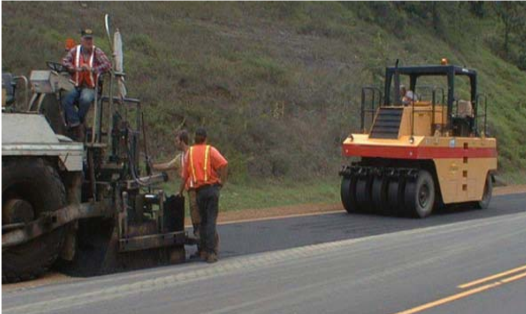
Figure 2-4 Rolling of Thin HMA Overlay (Newcomb, 2009)
