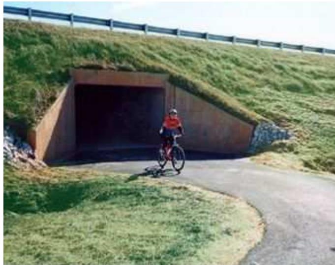
Figure 1.4: Picture of an Underpass Beneath a Four-lane Highway with High Traffic Volume
