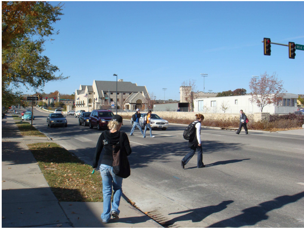
Figure 3.2: Picture of the Signalized Mid-block Crossing on Anderson Avenue.
