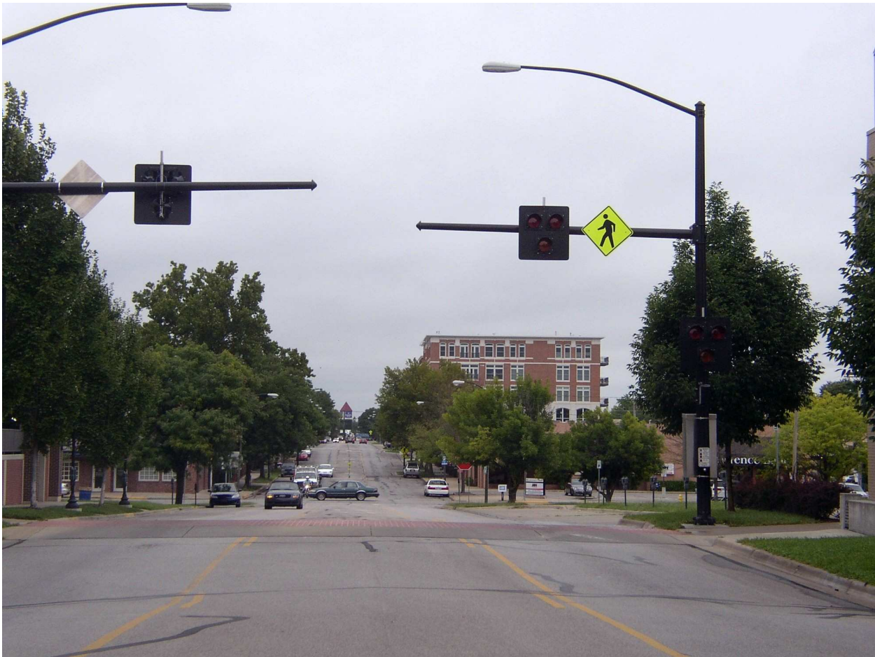
Figure 5.3: Photo of a Pedestrian Hybrid Beacon on New Hampshire Street, Lawrence, Kansas
