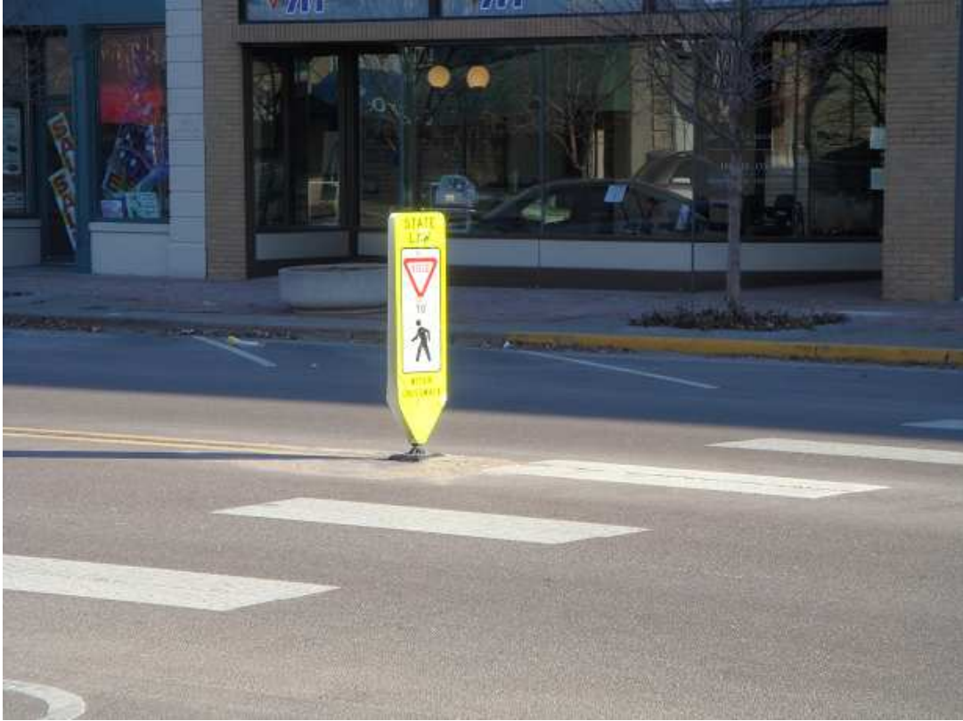
Figure 3.11: Crosswalk with In-Roadway Sign on Poyntz Avenue
