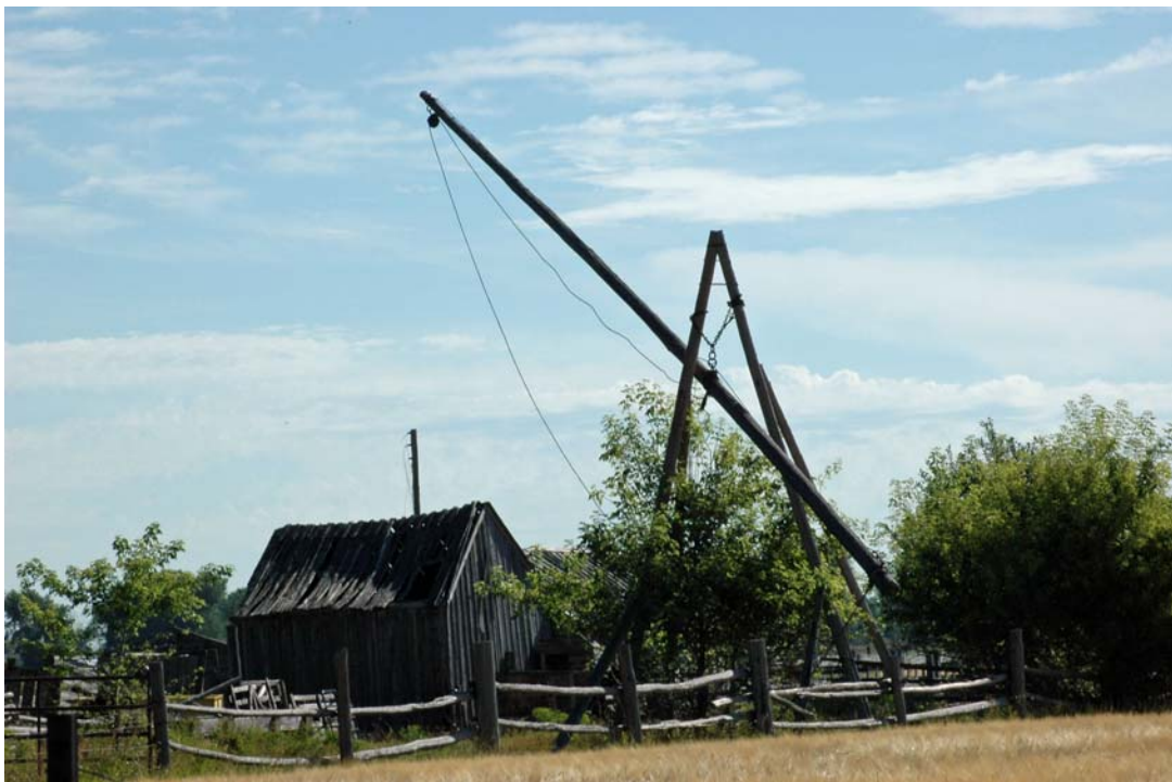
Figure 12. Chain/Hung Boom hay derrick near Idaho Falls, Idaho. August 2009. Photo: Linnea C. Sando.
