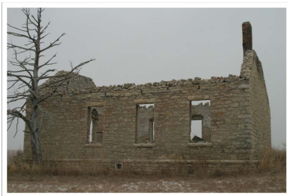
Figure 3. Ruins of the Former Bean School. Alma, KS. After a recent fire, only the stone outer walls of the school remain.
