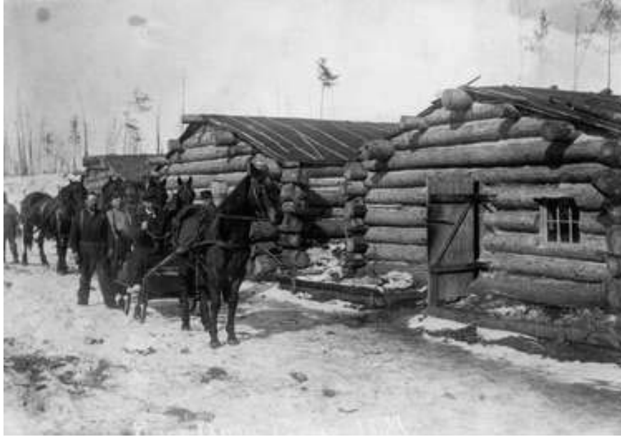
Figure 2.9: A typical early 20 th century logging camp cabin. Notice the small window on the house in the foreground. According to Roy and Gladys Snyder, such windows were rare in the logging camps and considered a luxury (Photo from Minnesota Forest History Center website).
