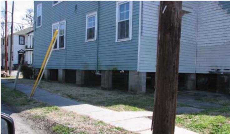
Figure 5.18 Elevated Home in Broadmoor Neighborhood
