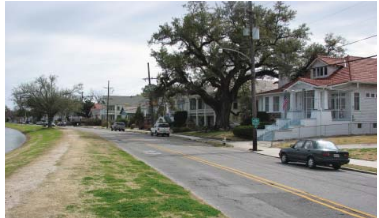
Figure 5.21 Mowed Banks Between Canal and Street.
