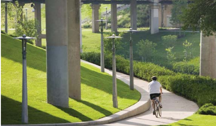
Figure 3.10 Lighting Under Interchange
