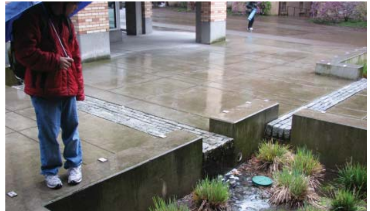
Figure 3.3 Portland Gutter Detention Basin
