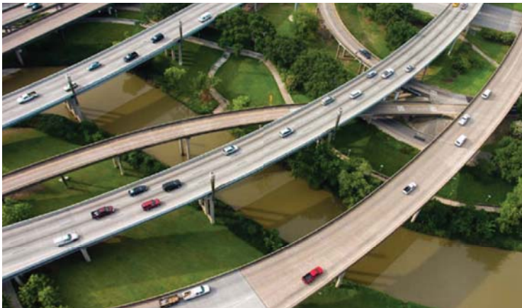
Figure 3.8 Overhead View of Bayou Under Highways
