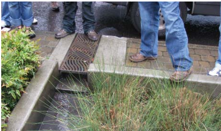
Figure 4.7 Permeable Planter Showing Curb Cut
