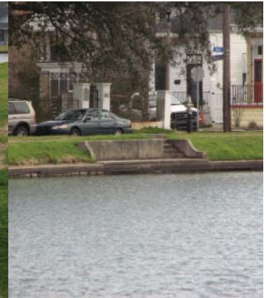
Figure 4.6 Concrete Steps Along Canal
