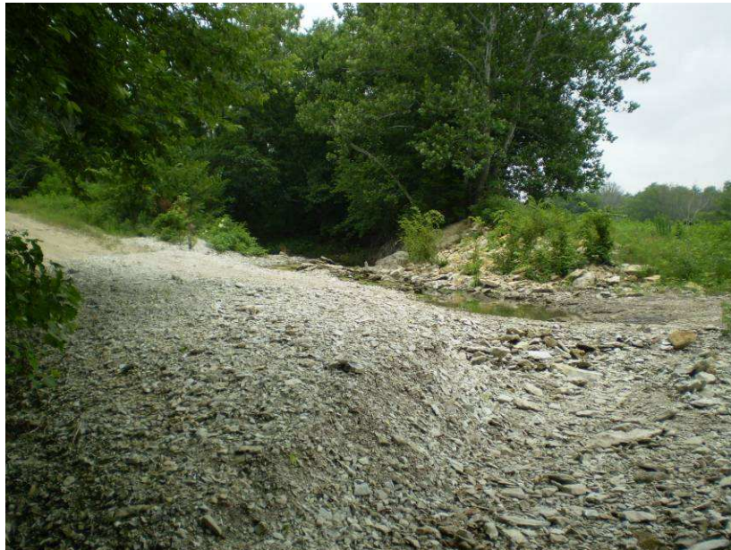
Figure 4-7. Sediment bar deposited on road at a stream crossings site, upstream view.
