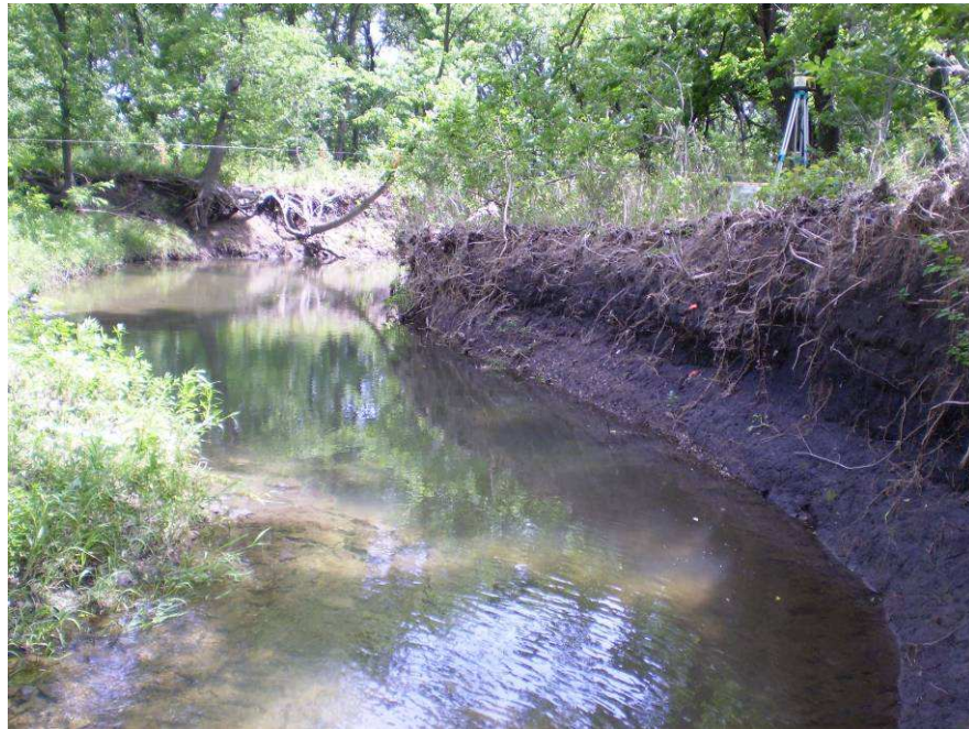
Figure D-13. Cross section transect 3 (pool) at Wind Creek, upland reach, downstream stream view.
