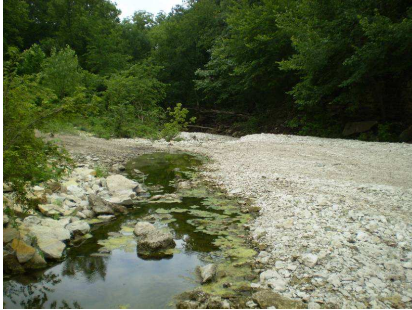
Figure 4-8. Sediment bar deposited on road at a stream crossings site, downstream view.
