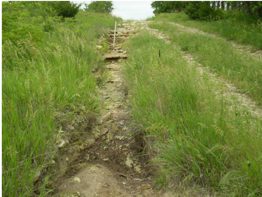
Figure 2-19. Gully forming on a road leading to stream crossing site.
