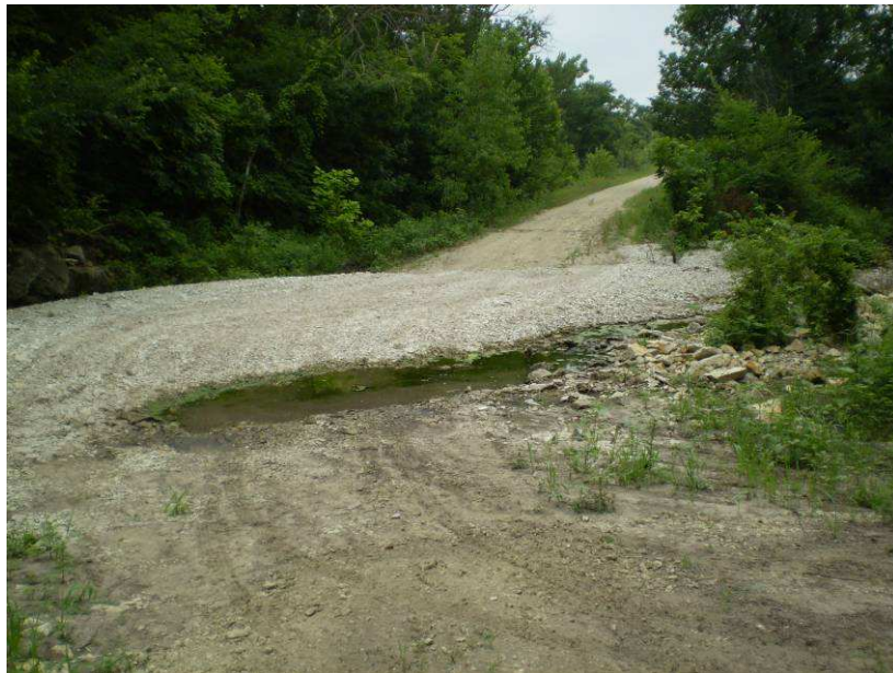
Figure 4-9. Sediment bar deposited on road at a stream crossings site, a view from left bank to right bank.
