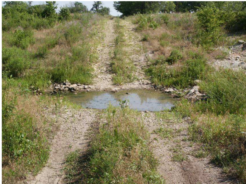
Figure 4-5. Wind Creek lowland stream crossing site, before May 05, 2007 flood event.
