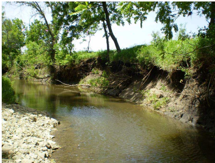
Figure F-7. Cross section transect 2 (pool) at Wind Creek, lowland reach, downstream view.
