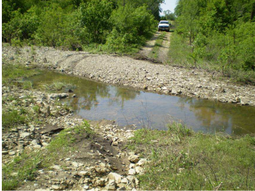
Figure 4-6. Sediment deposited on road at Wind Creek lowland stream crossing site, after May 05, 2007 flood event.
