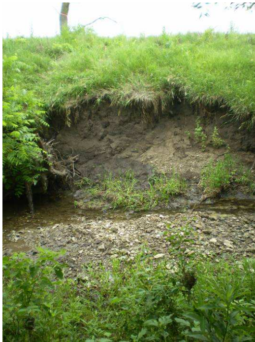
Figure E-20. Cross section transect 12 (riffle), view from left bank to right bank at Wind Creek, midland reach.
