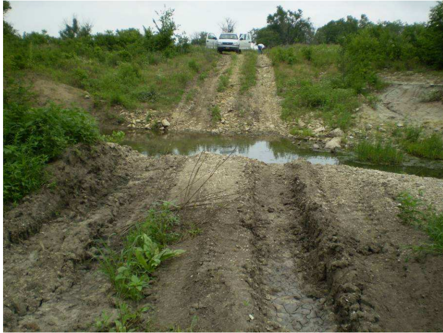
Figure 2-20. Approach roads can be a source of sediment.
