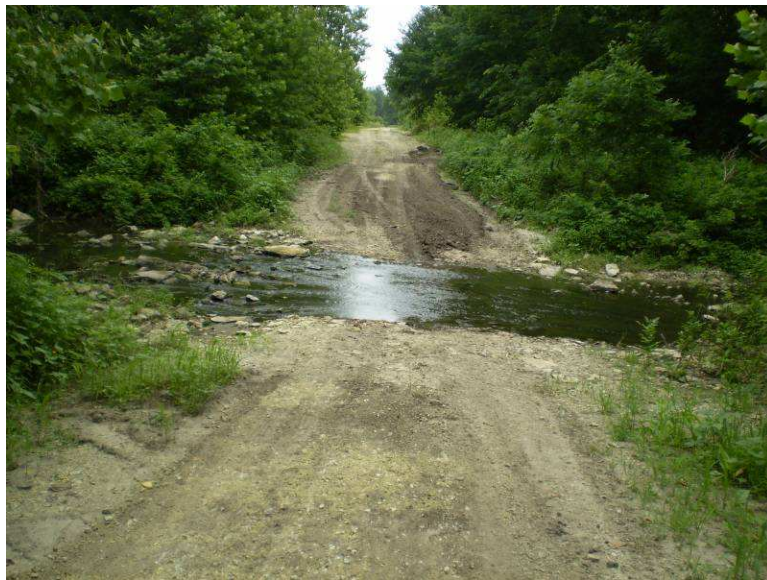
Figure 4-3. Properly functioning low water ford, located on a riffle.
