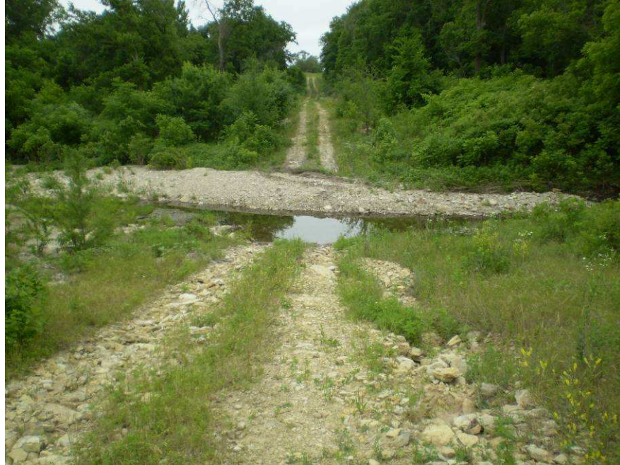
Figure F-8. Stream crossing, view from left bank to right bank at Wind Creek, lowland reach.
