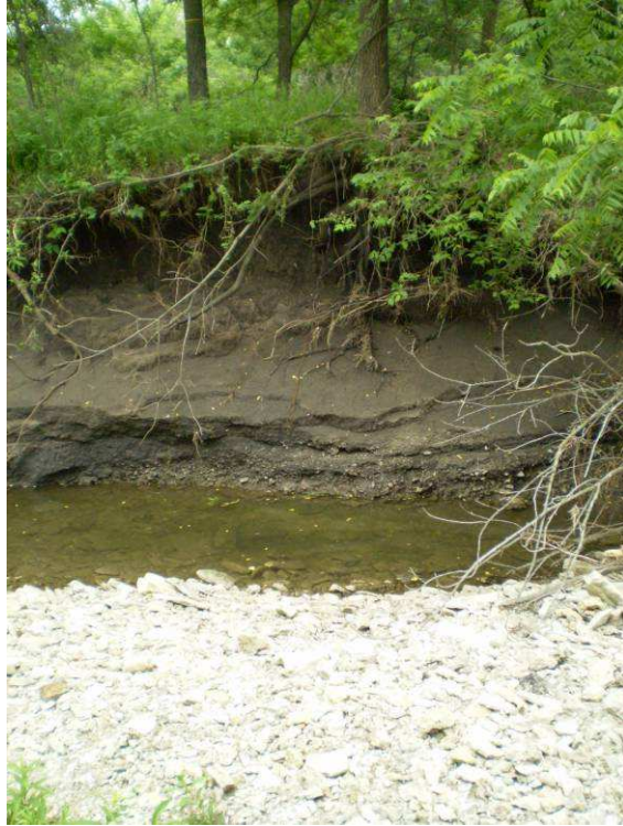
Figure F-14. Cross section transect 9 (run), view from left bank to right bank at Wind Creek lowland reach.
