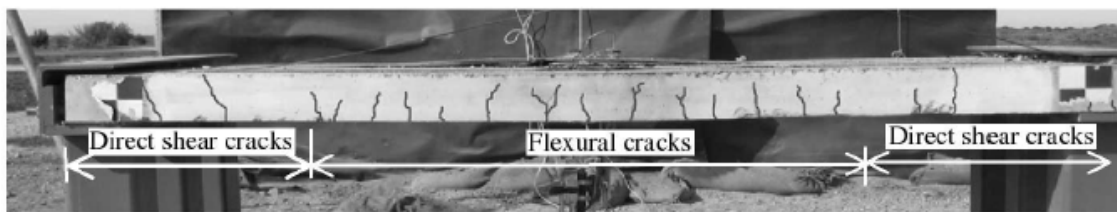
Figure 4.2-5 Crack pattern in RET-2 (Wu, Oehlers, Rebentrost, Leach, & Whittaker, 2009)
