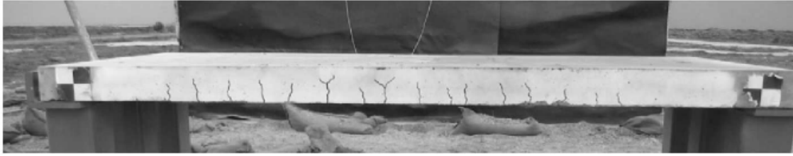
Figure 4.2-4 Cracks in specimen NRC-4 (Wu, Oehlers, Rebentrost, Leach, & Whittaker, 2009)
