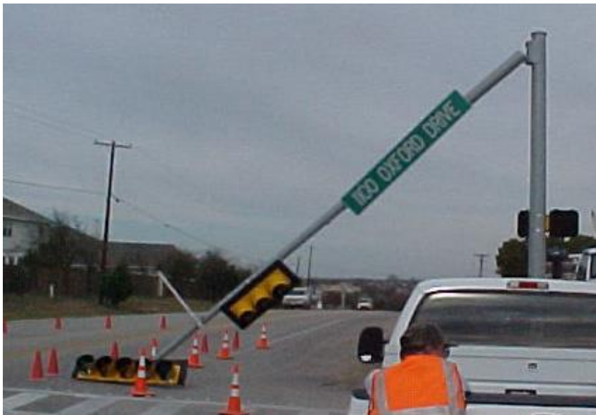
Figure 1-1 Falling cantilevered highway sign structure (Florea et al. 2007).
