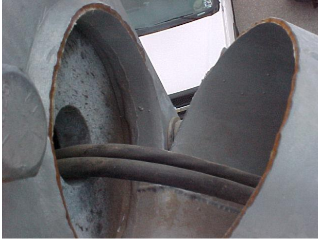
Figure 1-2 Fatigue failure at mast arm connection of traffic signal (Florea et al. 2007).
