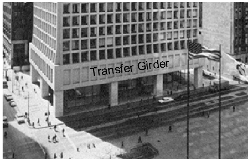
Figure 3.1 - Deep Beam, Brunswick Building, Chicago; picture courtesy of (columbia.edu)
