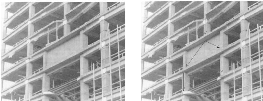
Figure 3.2 - Single Span Deep Beam; picture courtesy of (MacGregor & Wight, 2005)
