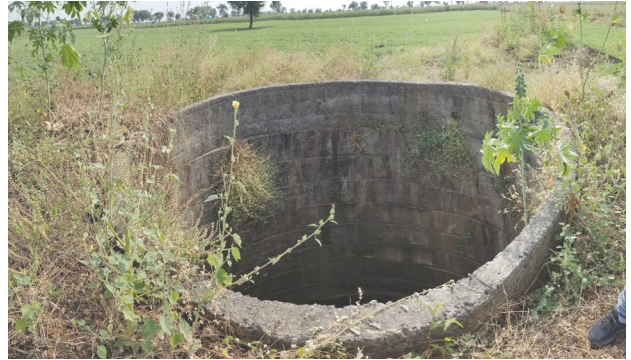
[56] Abandoned farm wells due to salty groundwater.
