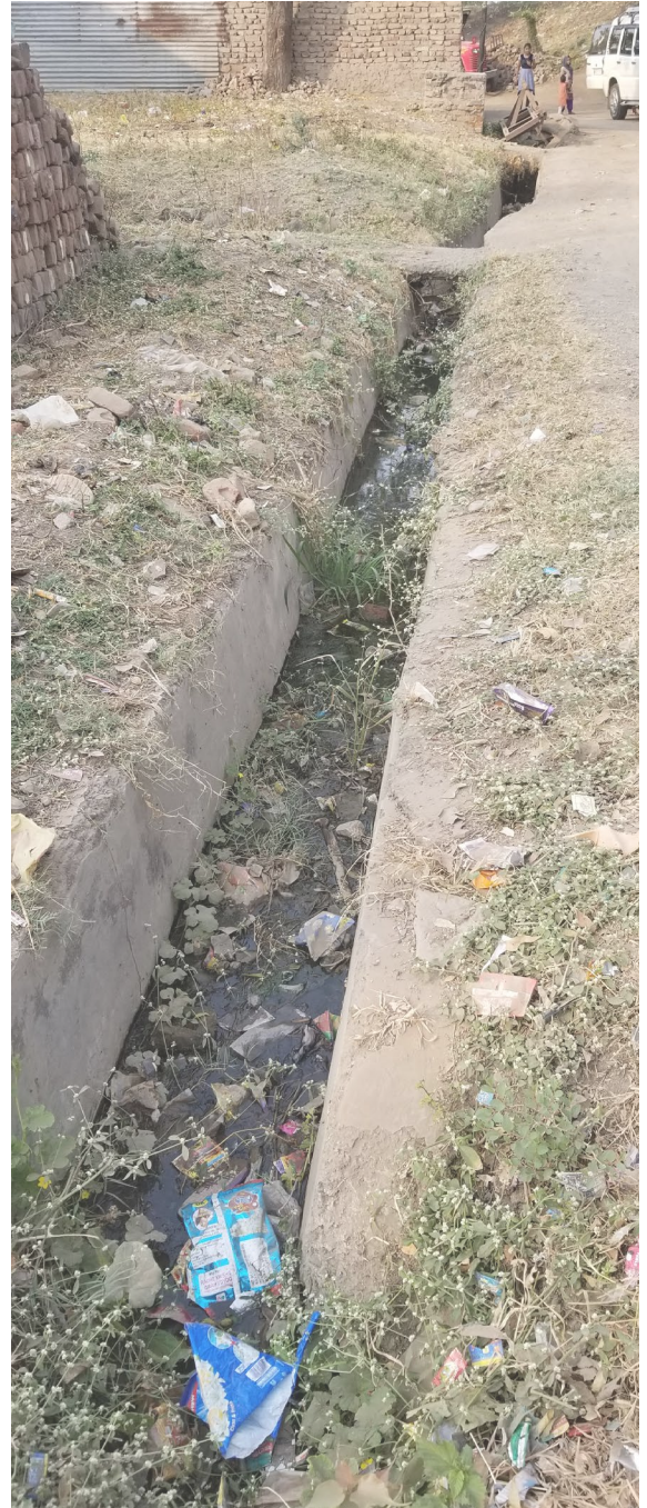
[55] Concrete nalli channel.
