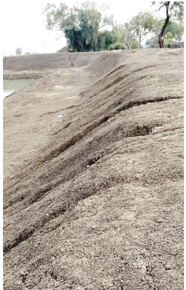
[52] Prominent soil erosion along the edges of the Talaab.
