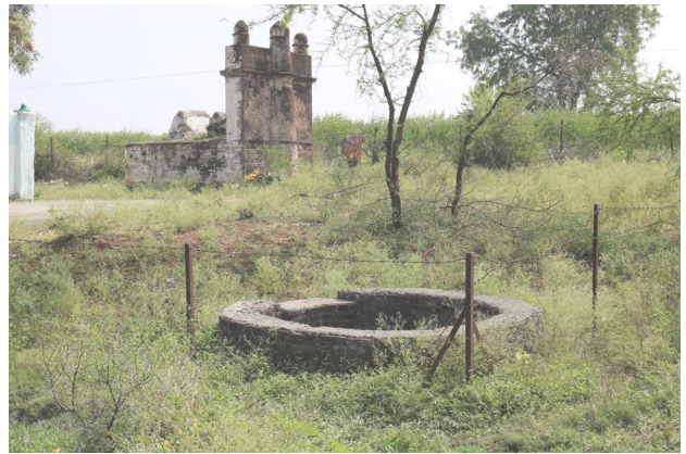
[57] Abandoned community well adjacent to the Mazaar.
