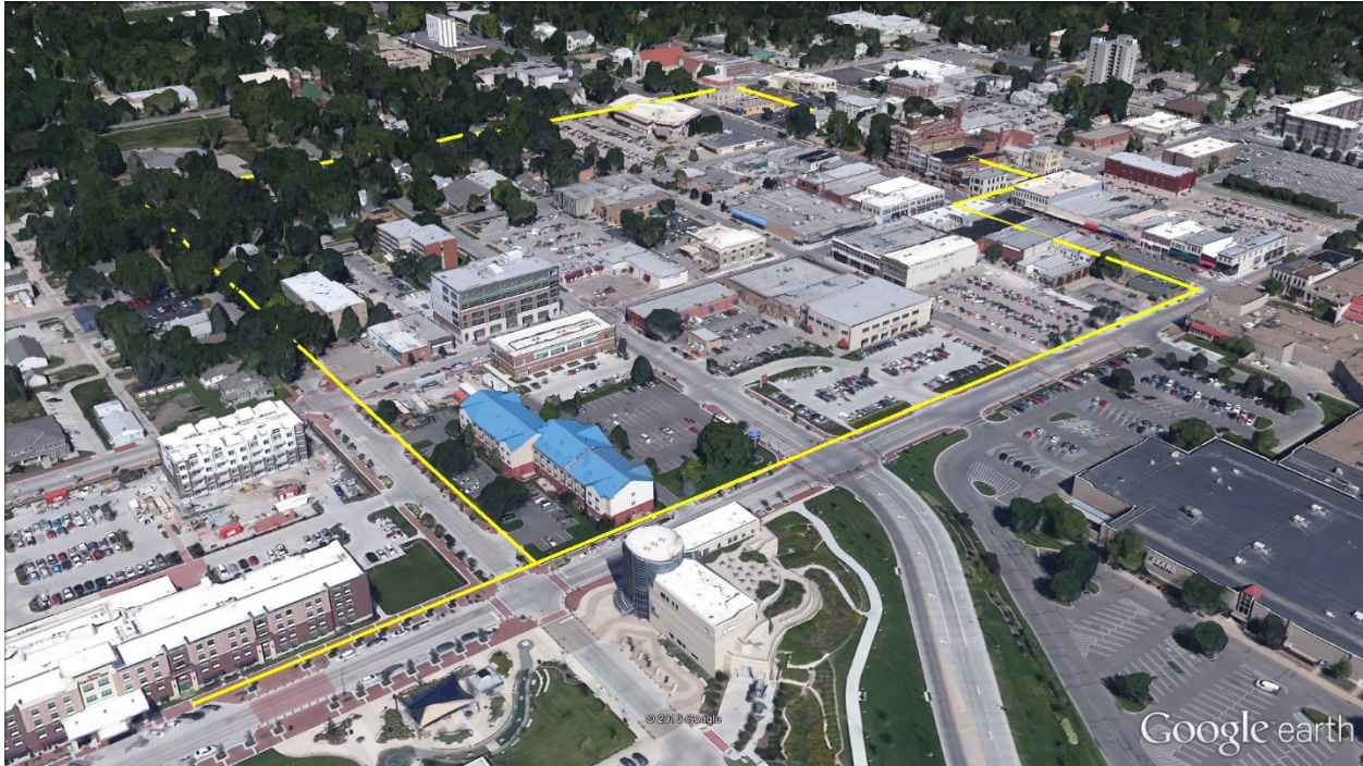
Figure 2 Site: Route (yellow line) in study area of Manhattan, KS (Image by Google Earth)
