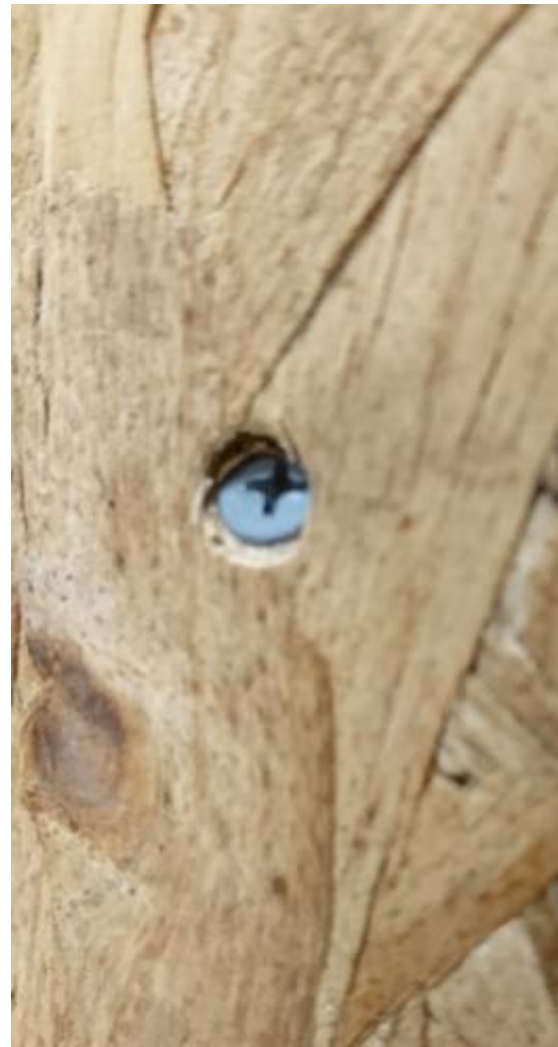
Figure 5-6 Screw Head after Failure
