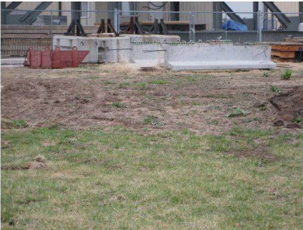
Figure 7-3 Picture of KOCE Site Before Construction, Showing Original Elevation
