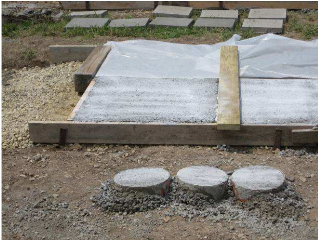
Figure 7-12 Plastic-Covered Curing and Curing Compound Applied
