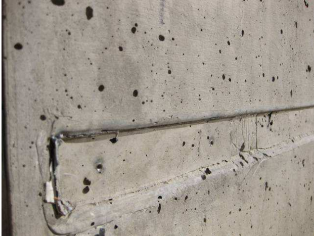
Figure 7-19 Inserts Embedded in the Concrete
