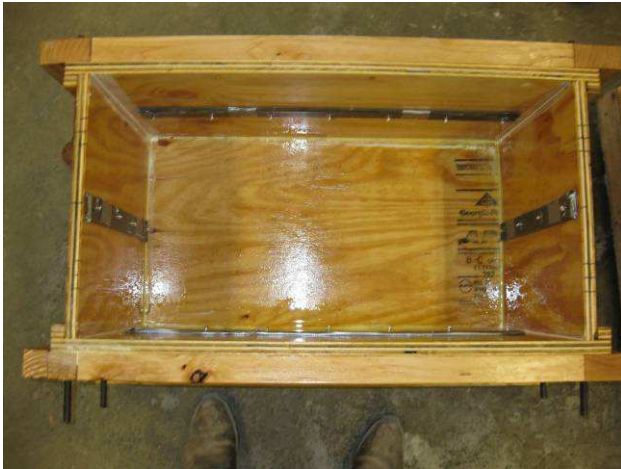
Figure 7-17 Steel Strips Bolted to the Forms
