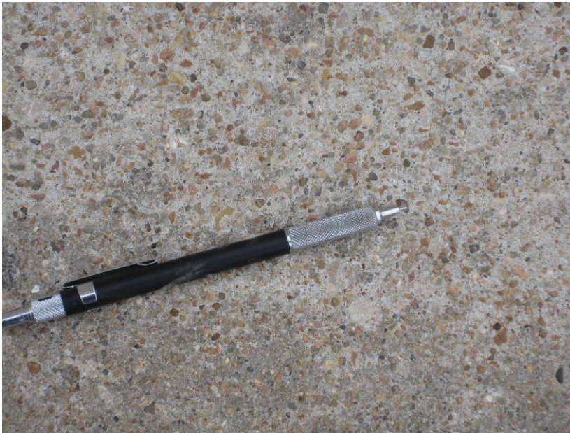
Figure 2-1 Severely Salt-Scaled Sidewalk
