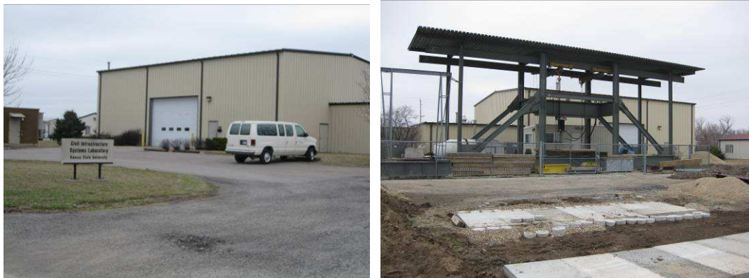
Figure 7-2 CISL Building and Load Frame
