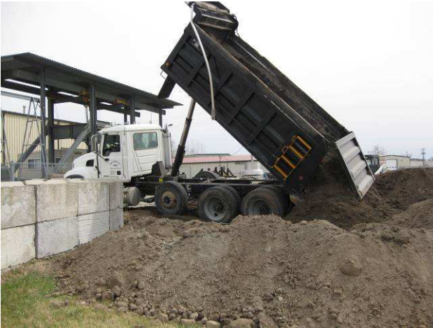
Figure 7-4 Local Contractor Delivering Fill
