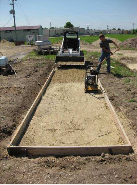
Figure 7-6 Compacting AB3 Inside of Formwork
