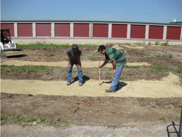
Figure 7-5 Using Water Level to Check Elevation
