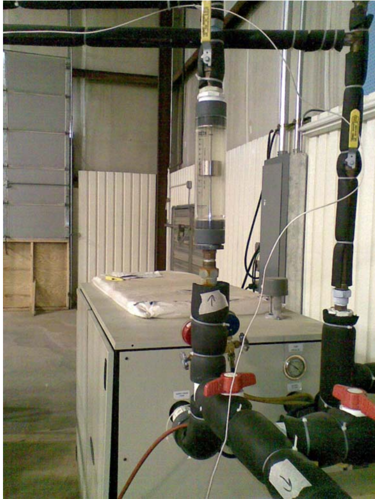
Figure A-3 Chiller Flow Meter
