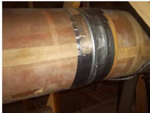
G) Supply Duct Joint
