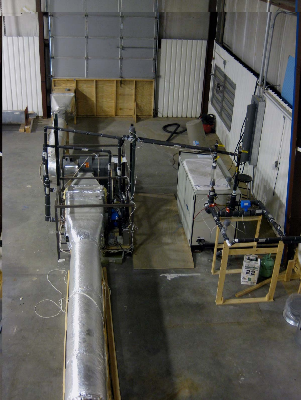
Figure 3-10 A View of the Air Supply Heating & Cooling System Installation
