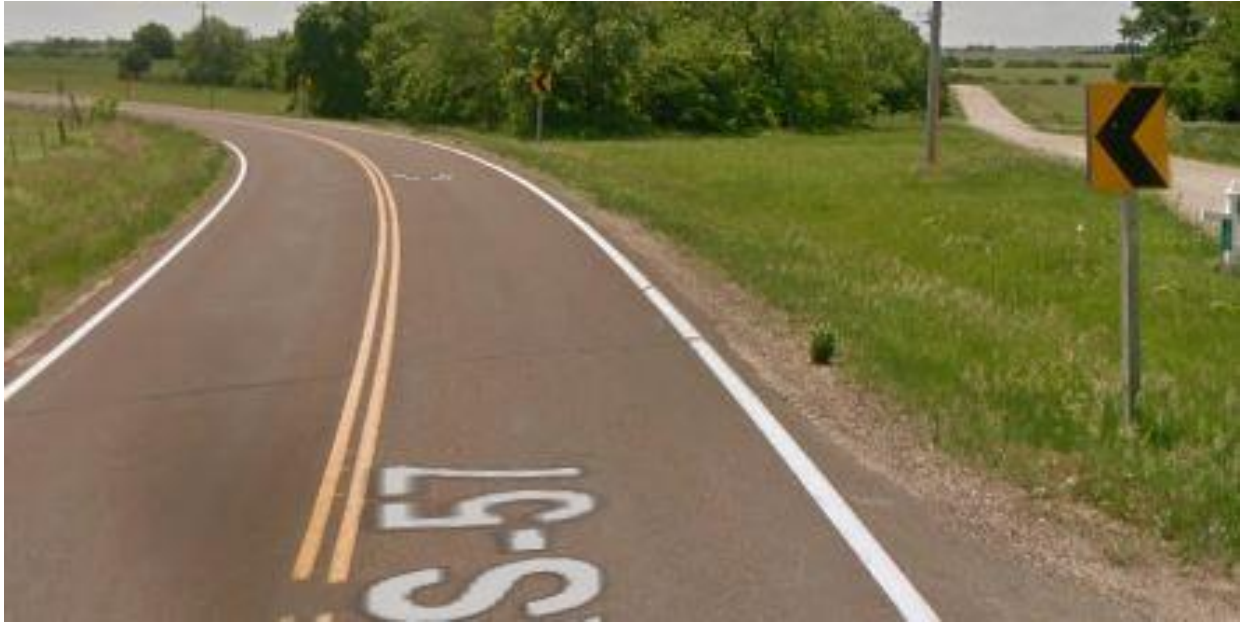
Figure 2.3 Chevrons on rural two-lane undivided curved road segment
