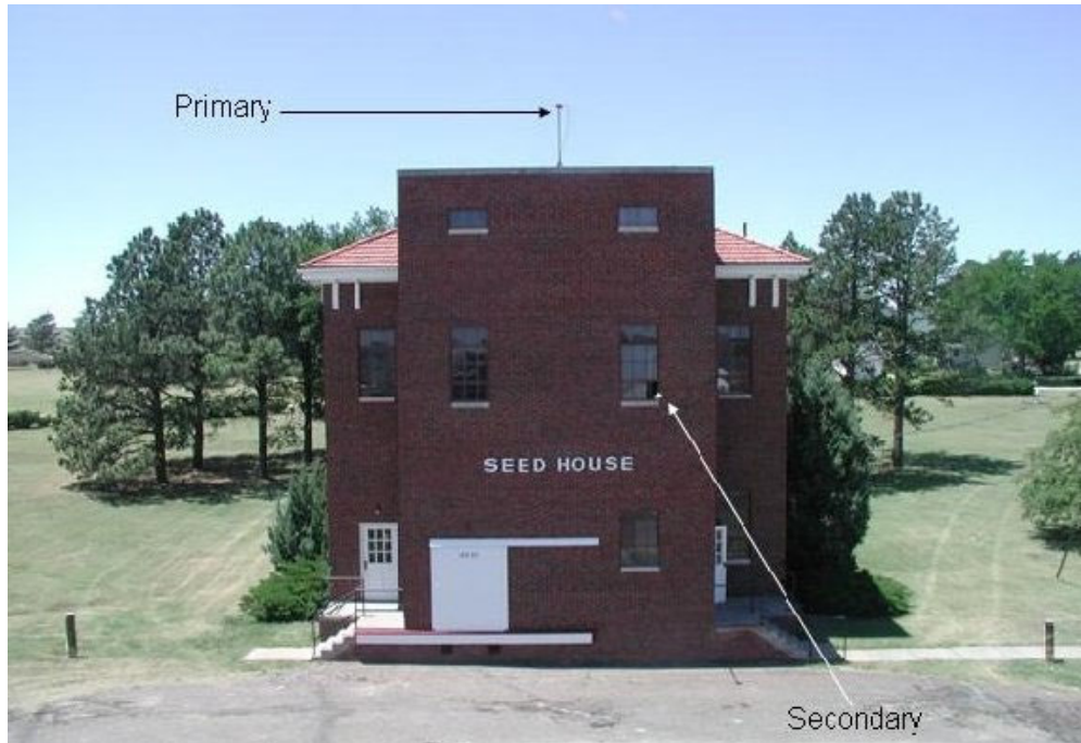
Figure 1-2. Deployment of primary (roof top) and secondary (window) GPS antennas for the static test. Building faces east.
