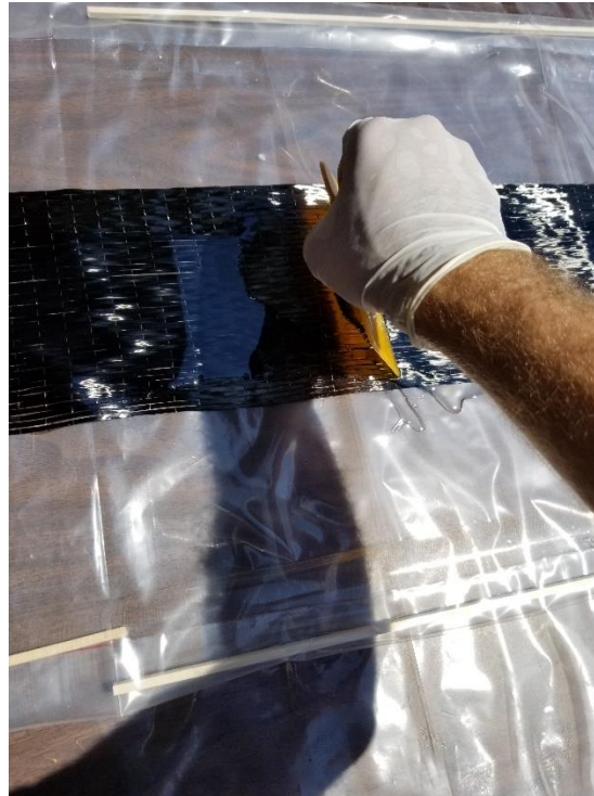
Figure 10. Saturating the carbon fibers with neat resin
