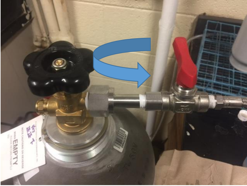
Figure A-6 CO 2 cylinder switch on
