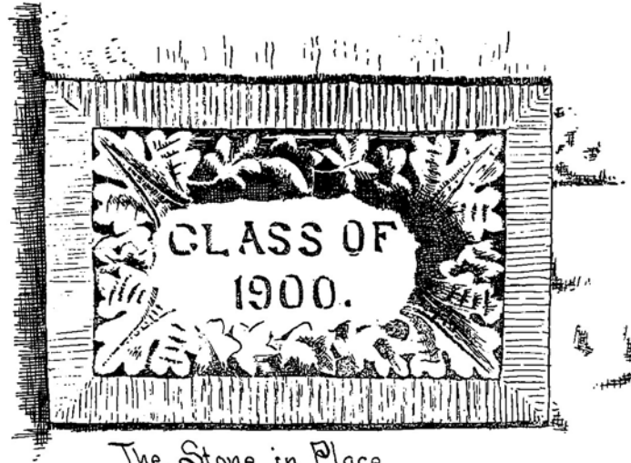
The Stone in Place
