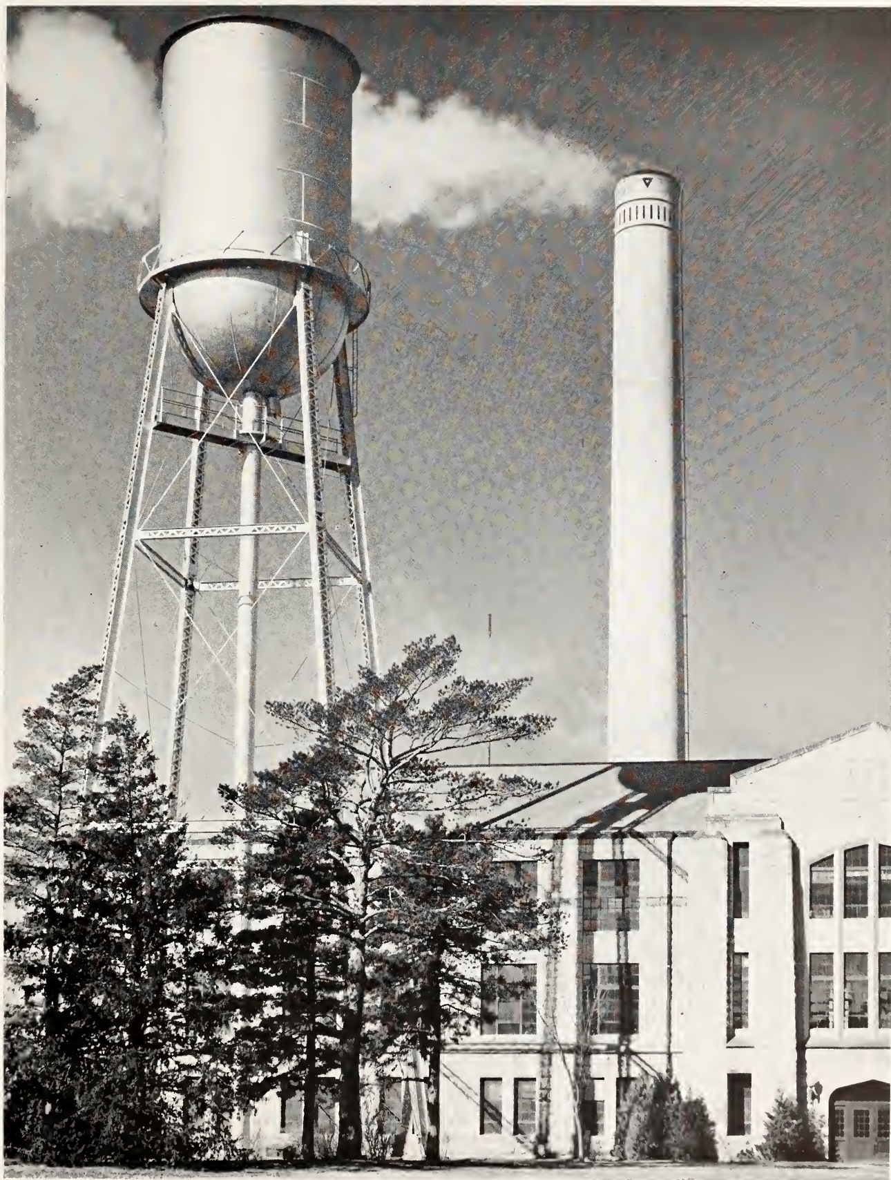
IN THE POWER PLANT is the electrical equipment controlling the ringing of class bells and the blowing of whistles.
