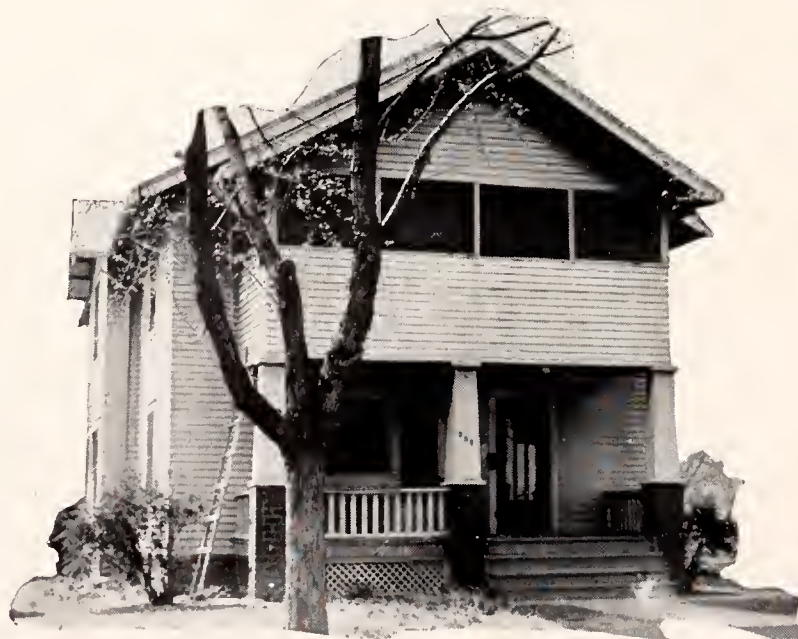
351 NORTH FIFTEENTH STREET
