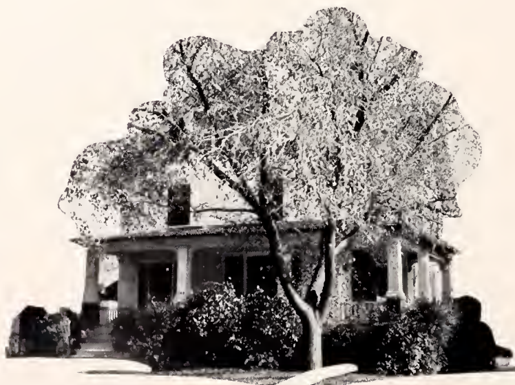
340 NORTH SIXTEENTH STREET
