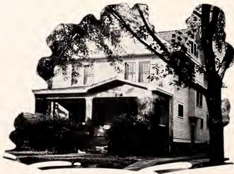
303 NORTH SIXTEENTH STREET
