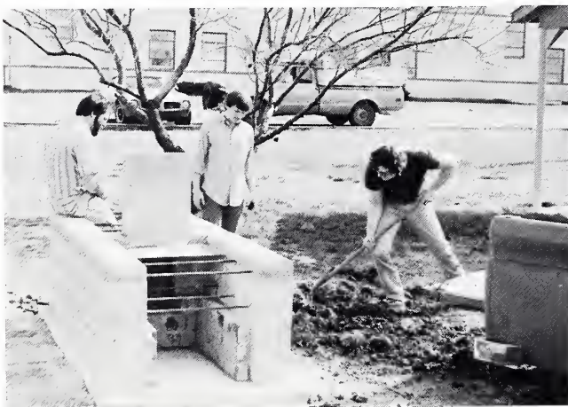
Bill Rutz and Richard Williams provide guidance while David Jones does the heavy work with the shovel.
