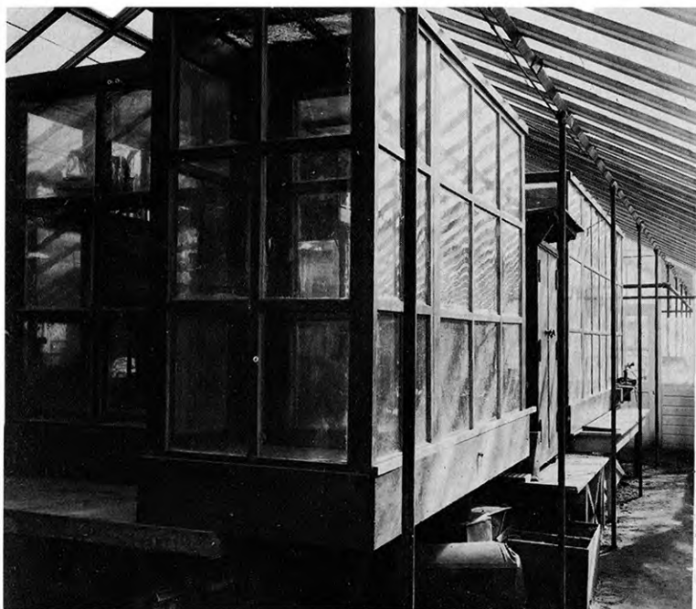
The breeding chamber of the first K. S. A. C. air-conditioned insectary (left) and the massive machinery used to produce controlled temperature and humidity. The chamber was double-glassed walled, 6' wide, 8' long, 7' high. It was very crude and insufficient compared to present environmental control insectaries at K-State.
