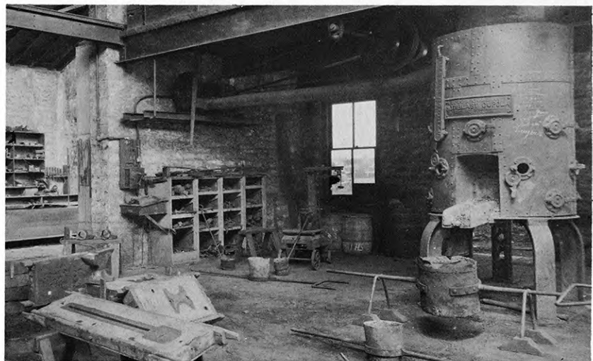
Foundry interior, an early photo.
