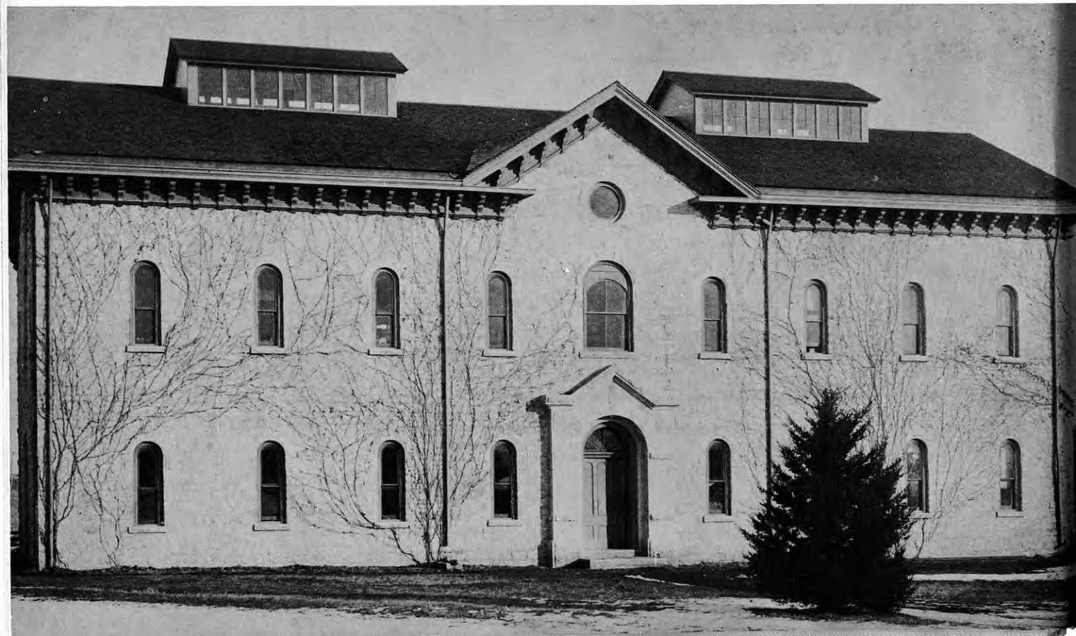
Barn—as constructed in 1873, was the west wing of the planned structure and became known as Farm Machinery Hall, also Farm Mechanics Hall.
