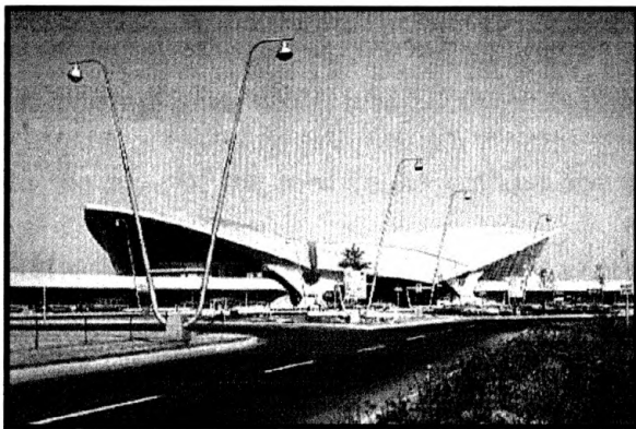
Figure 1.25: TWA terminal, main entrance (Stoller, 1999, p. 23)
