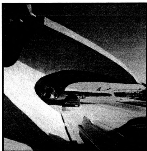
Figure 1.23: TWA terminal, main entrance (Stoller, 1999, p. 25)
